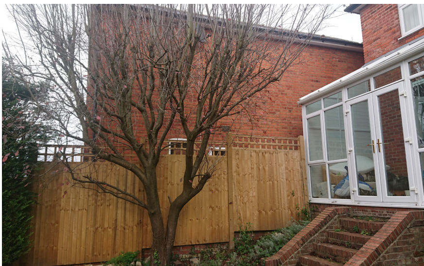
Fig. 4 - Flank wall of number 38 and existing conservatory of number 40
