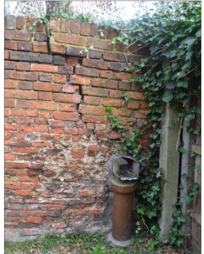
Figure 15 &16: Close ups of the southern section of the wall showing the various repairs with different mortar mixes, & significant structural crack
