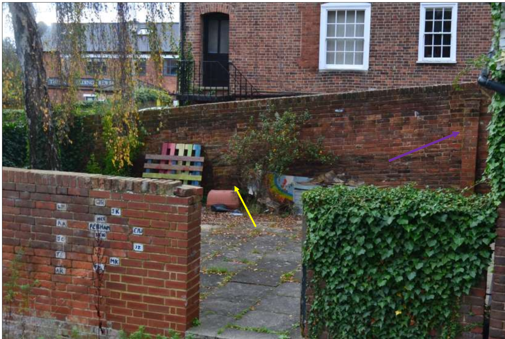
Figure 17: Rear of the southern elevation of the wall - note the full height buttress identified in purple and the low-level buttress in yellow
