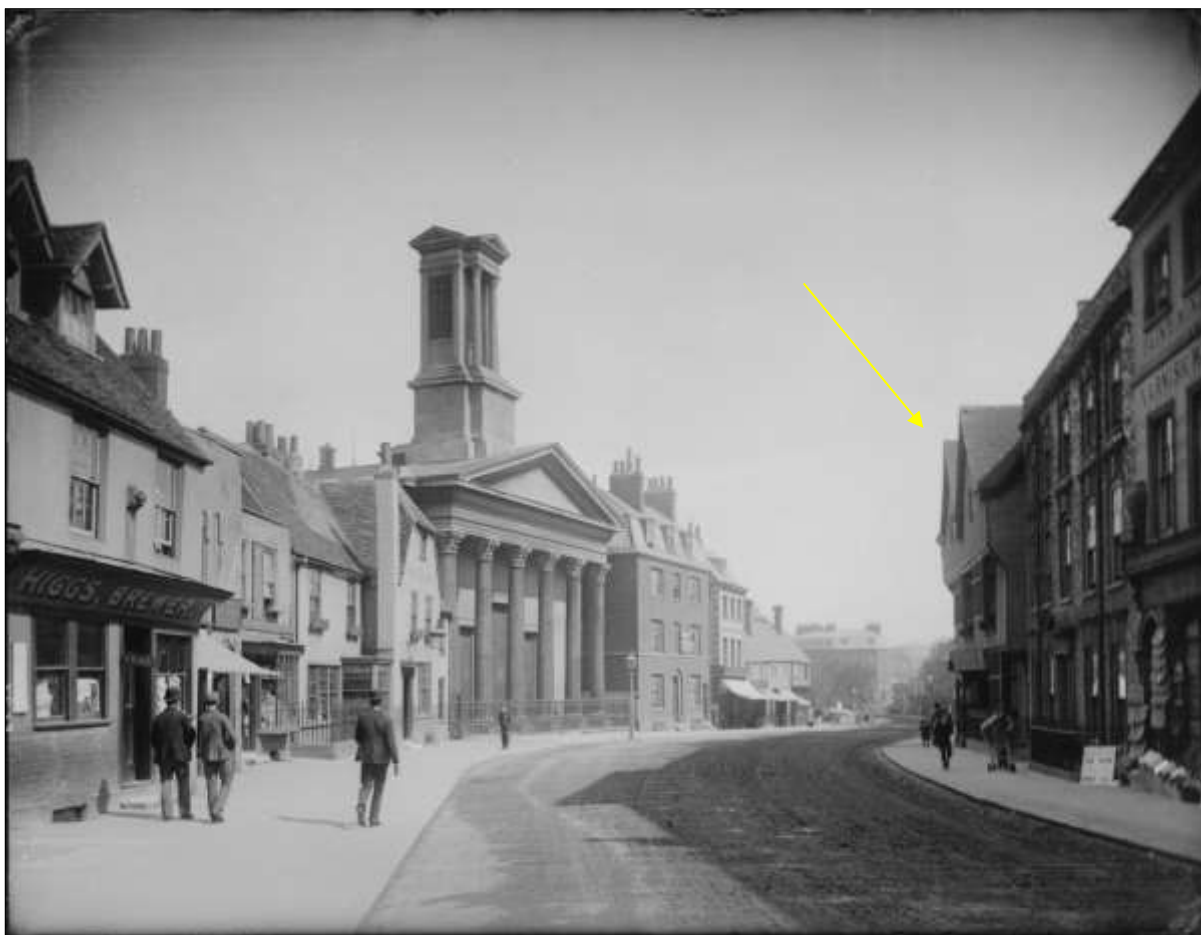
Figure 10: c.1890 photograph of Castle Street - note the width of the street. No. 17 is highlighted in yellow
