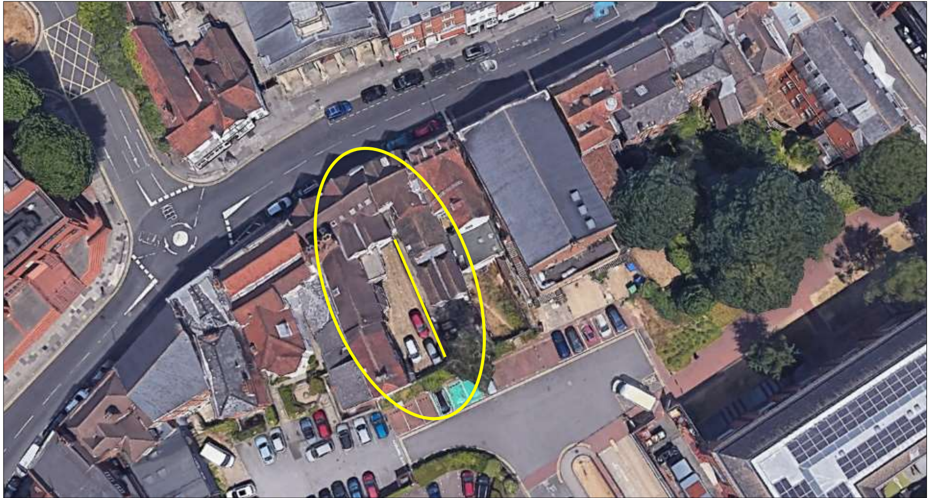
Figure 1: Brick wall to the rear of 17 Castle Street highlighted in yellow
