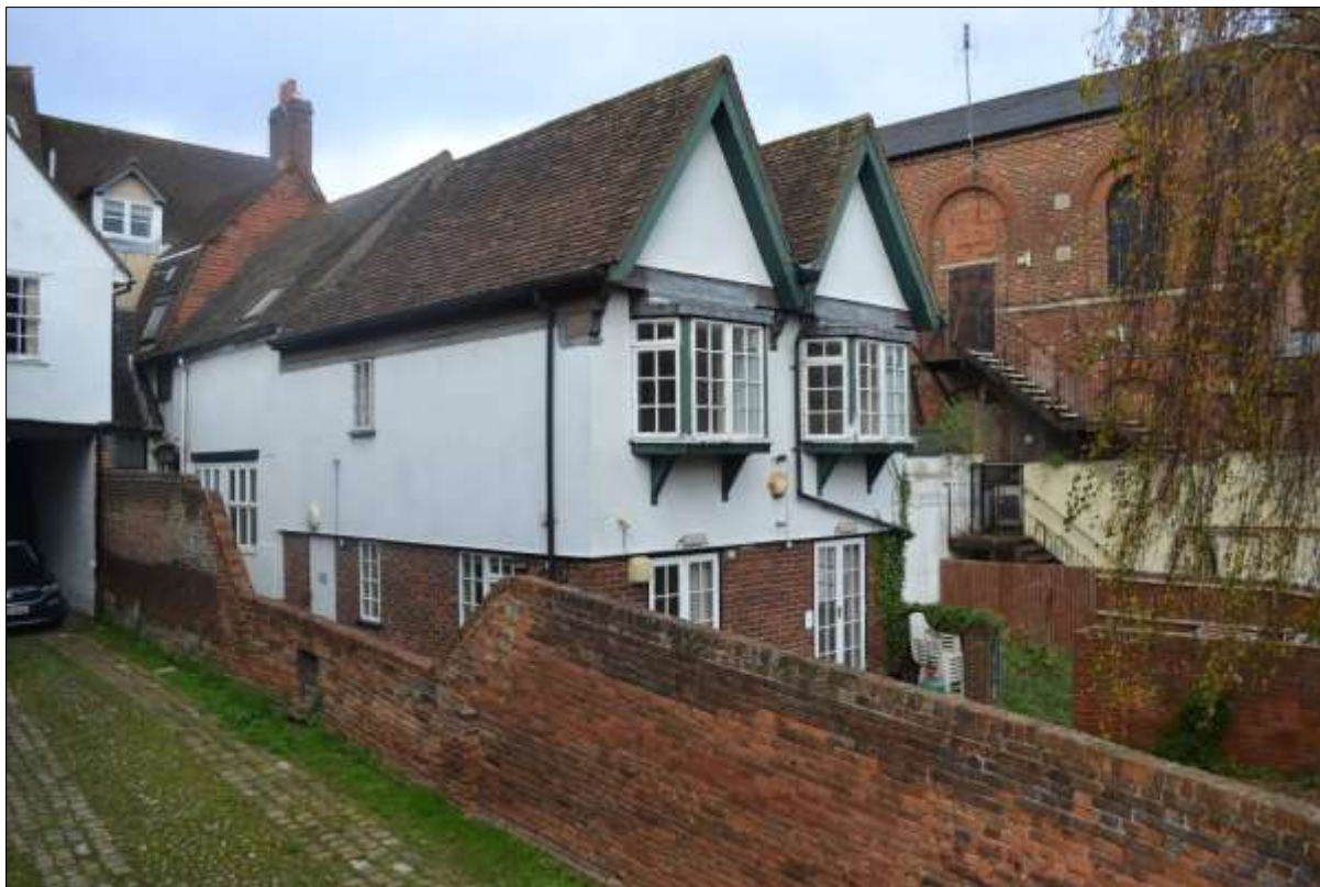
Figure 13: Brick wall to rear of 17 Castle Street
