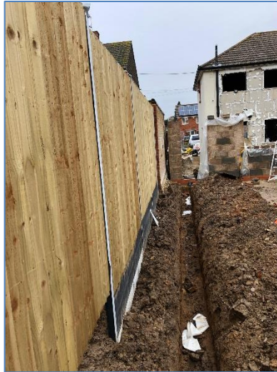
Fig 4. Site photo provided by agent on 20/11/2020.
