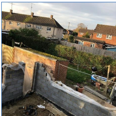
Fig 1. Site photo provided by agent on 25/11/2020.
