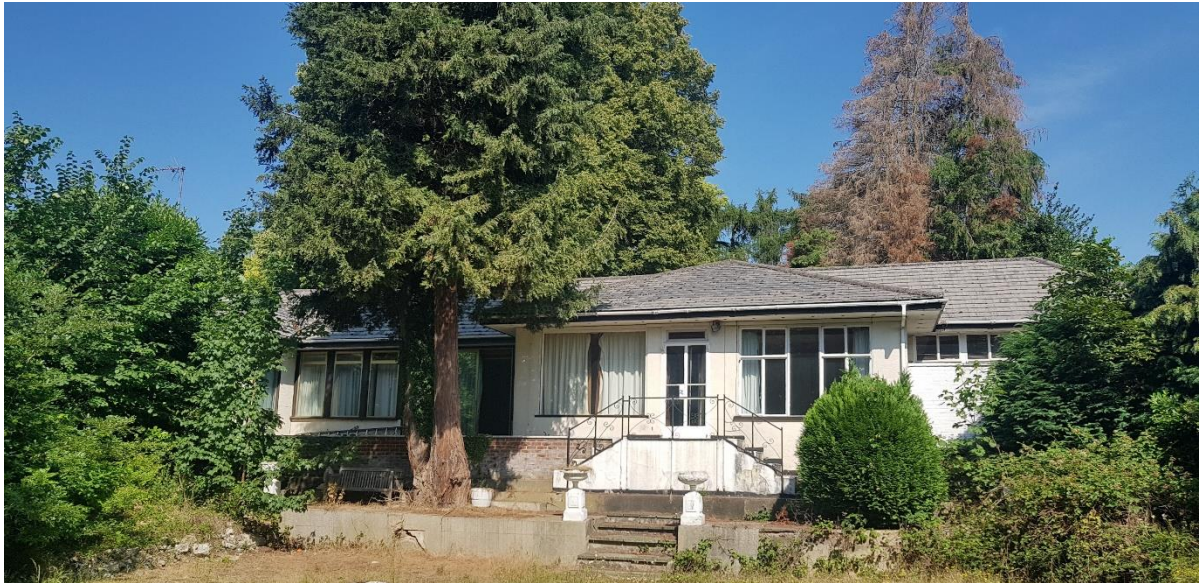
Figure 2: Photo of Existing Rear Elevation Facing North West
