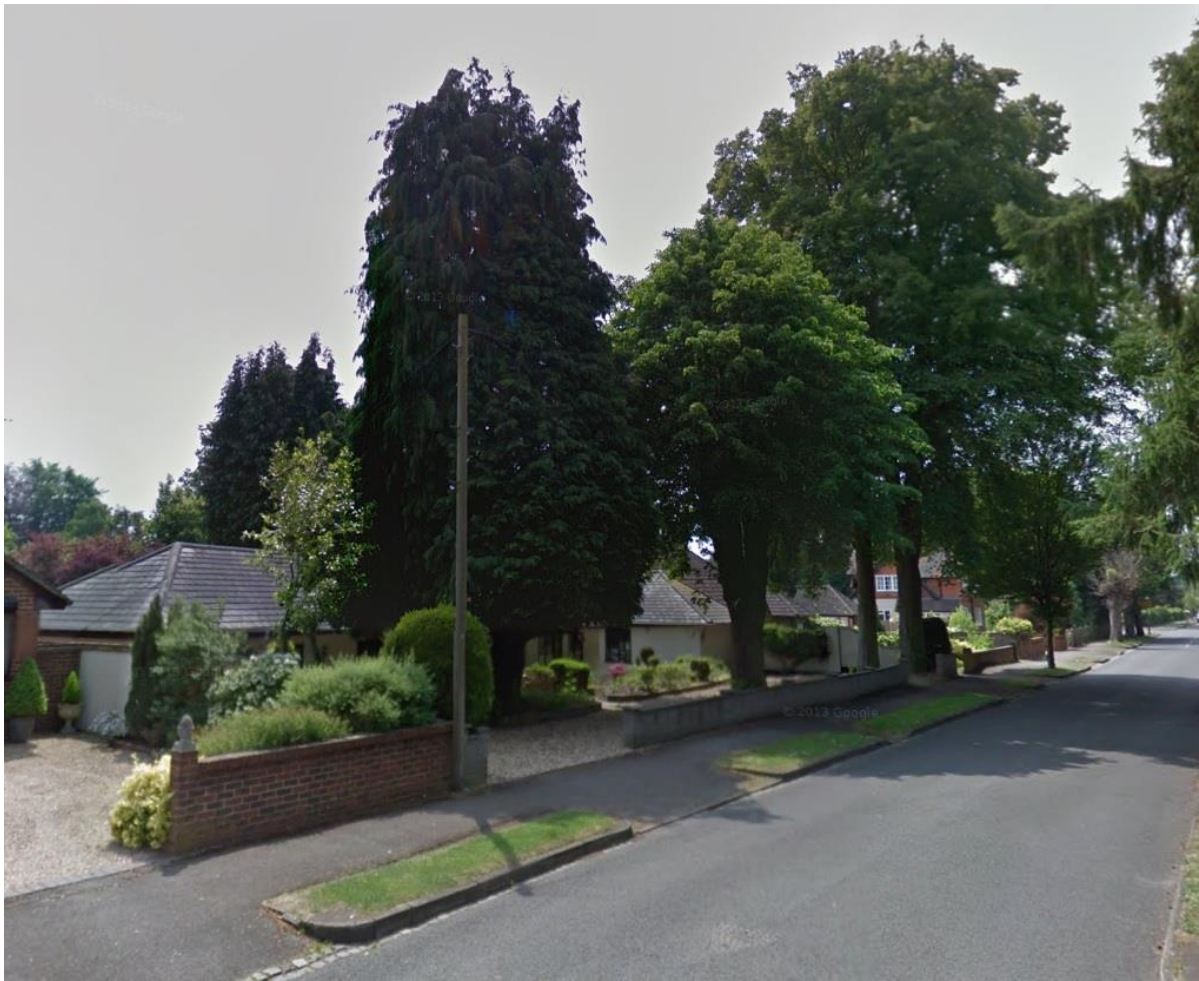
Figure 3: Photo of Existing Front Elevation Facing South East
