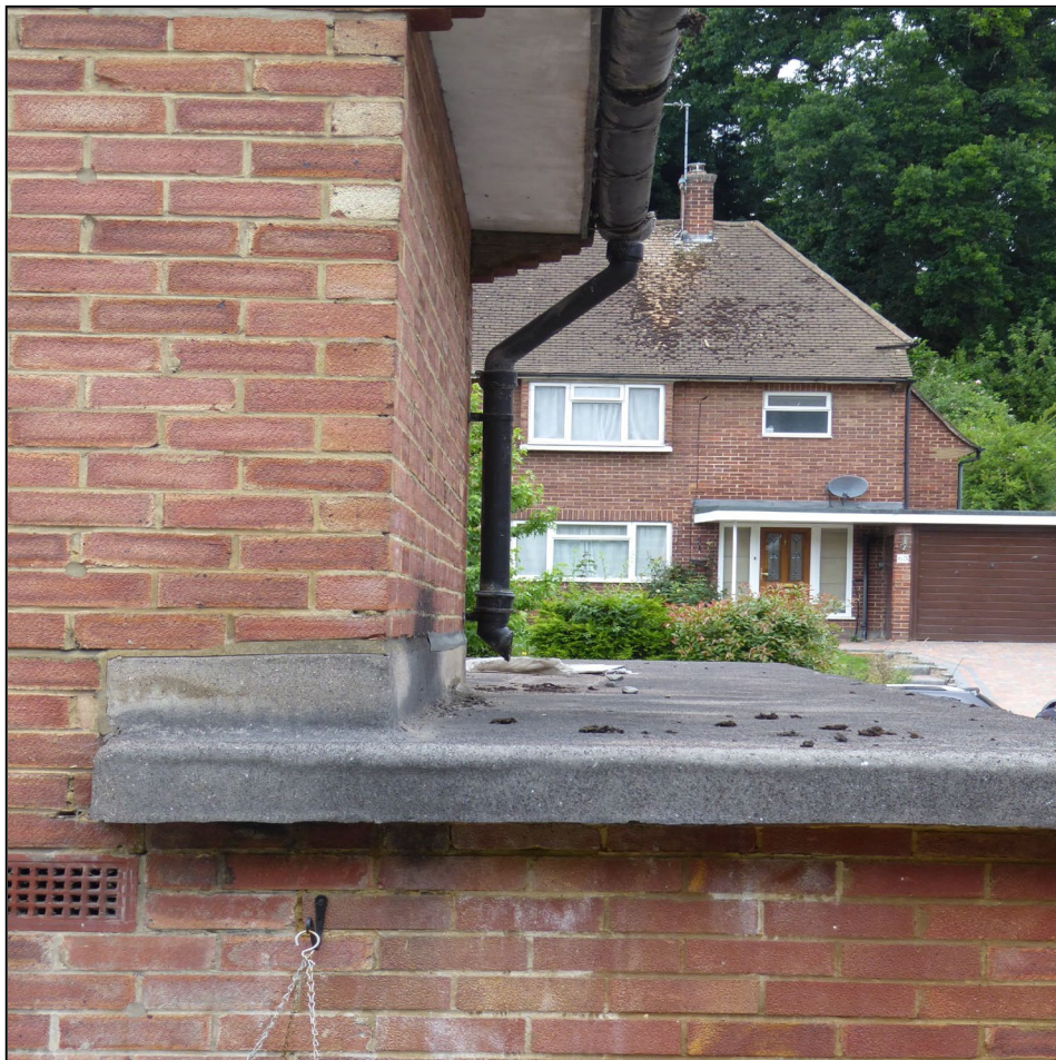
Figure 5. Example of flat roof on building. 60 Rotherfield Way, Reading. 30.06.20
