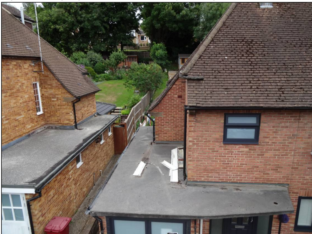
Figure 11. The garage roof. 60 Rotherfield Way, Reading. 30.06.20
