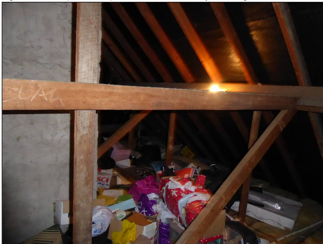
Figure 12. Example of loft space, 60 Rotherfield Way, Reading. 30.06.20
