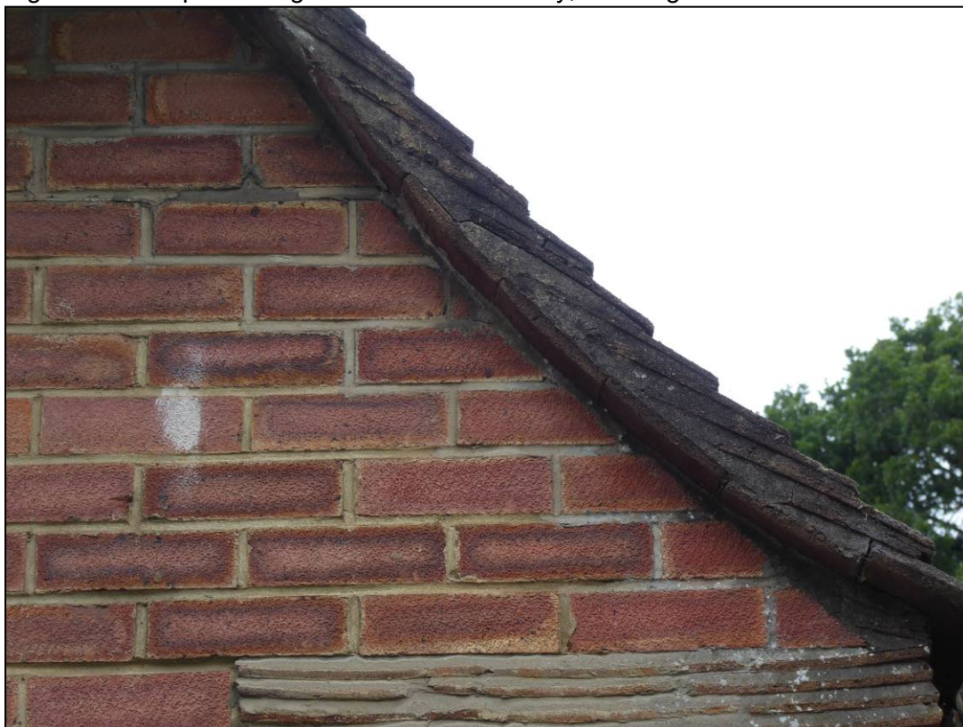
Figure 8. Example of verges. 60 Rotherfield Way, Reading. 30.06.20
