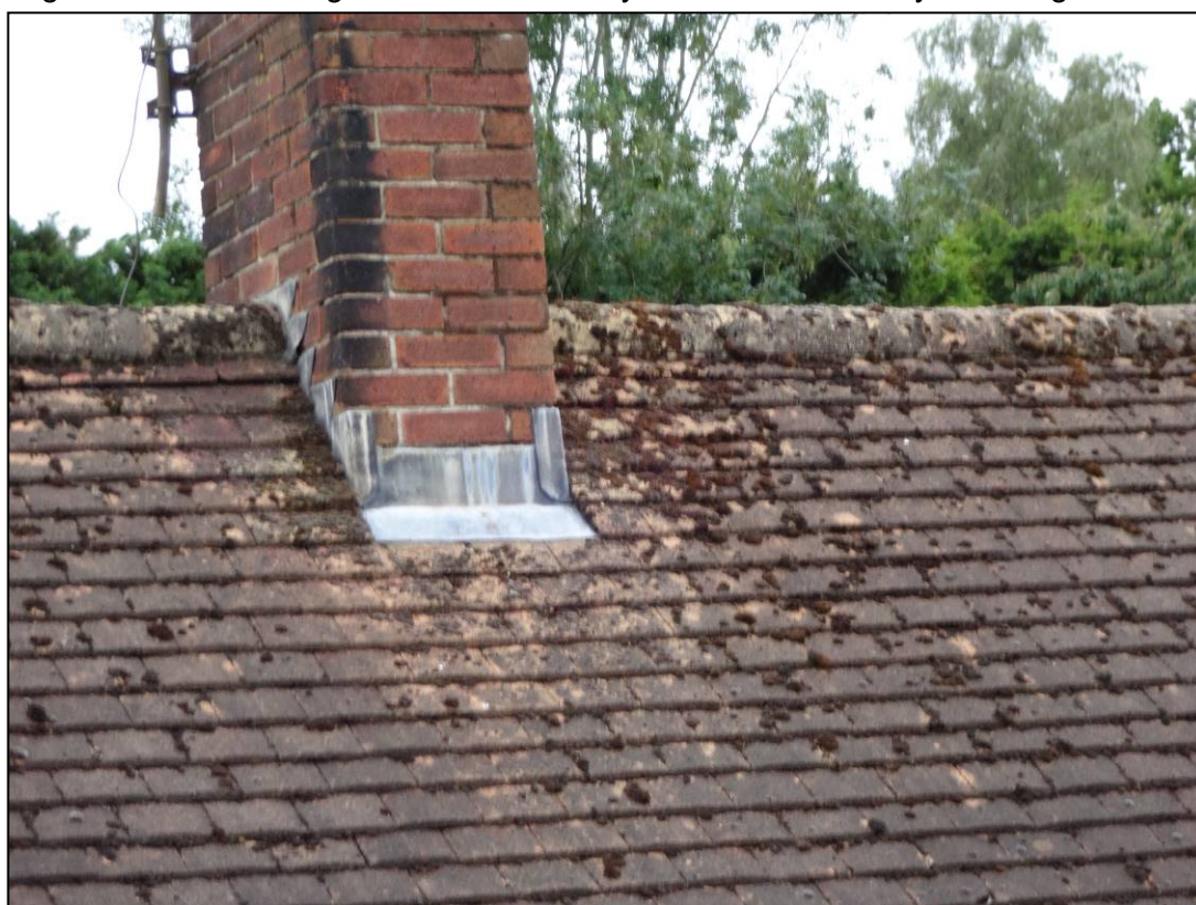
Figure 9. Lead flashing around the chimney. 60 Rotherfield Way, Reading. 30.06.20
