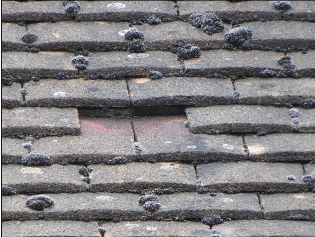
Figure 6. Single missing tile on building, 60 Rotherfield Way, Reading. 30.06.20
