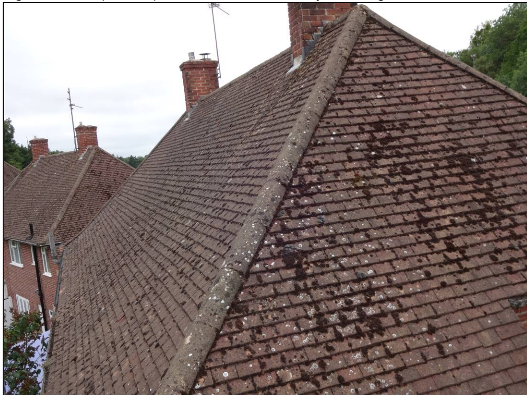
Figure 7. Example of hip tiles. 60 Rotherfield Way, Reading. 30.06.20
