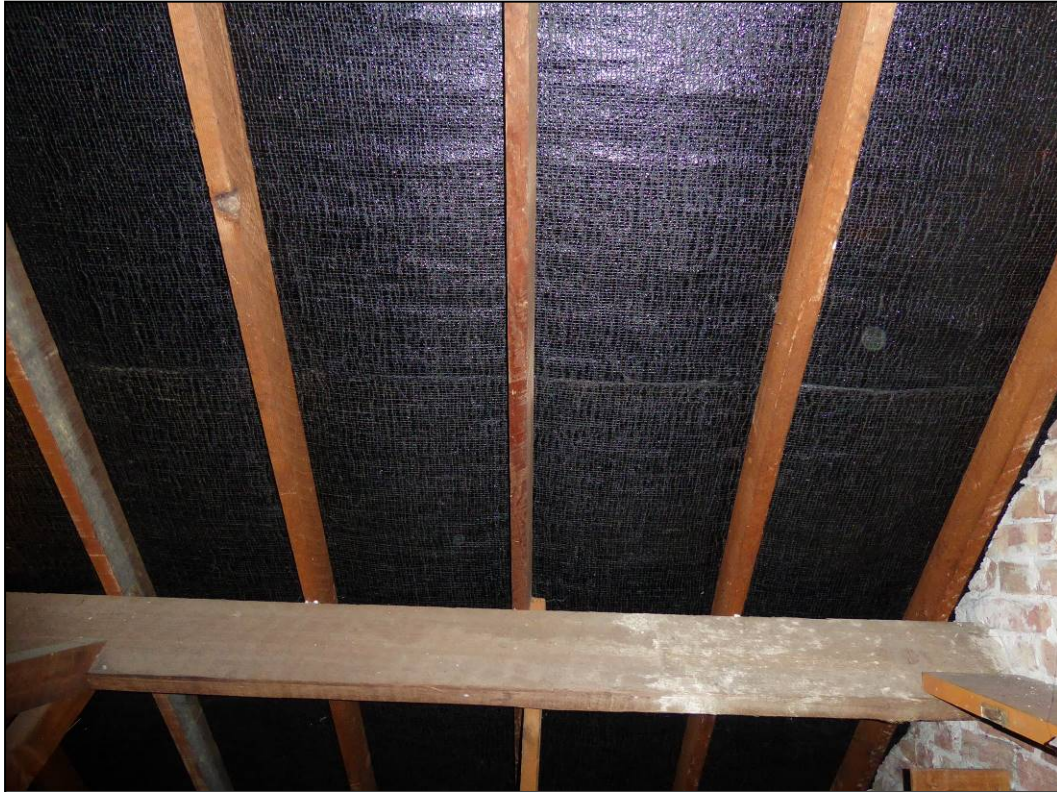
Figure 13. Example of bitumen lining. 60 Rotherfield Way, Reading. 30.06.20
