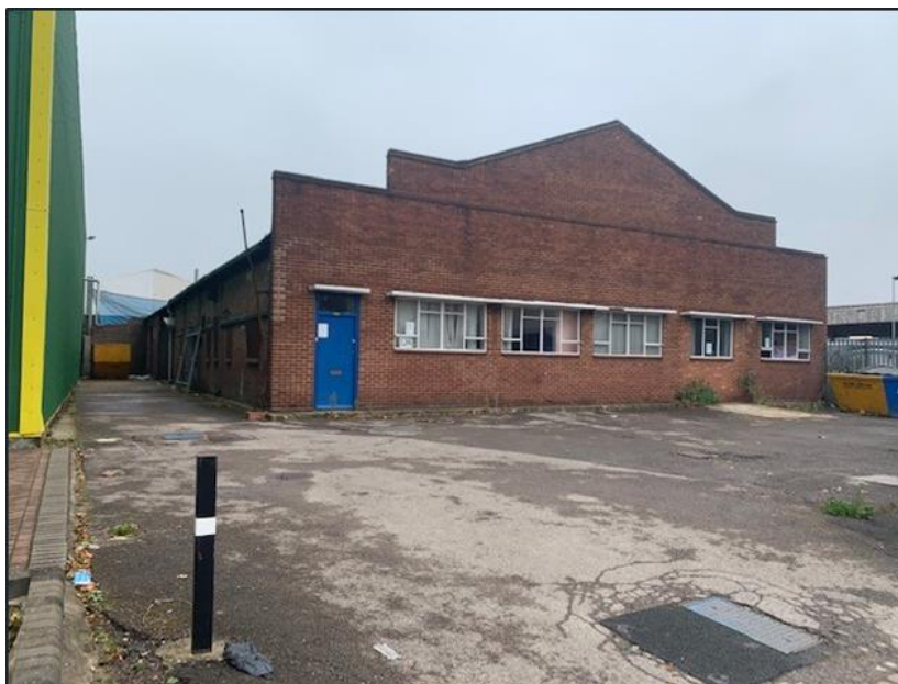
No. 124 Cardiff Road (Application Site - former UPS Depot and is currently vacant)
