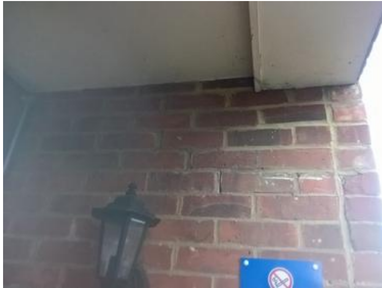
FIGURE 03 External Damage
