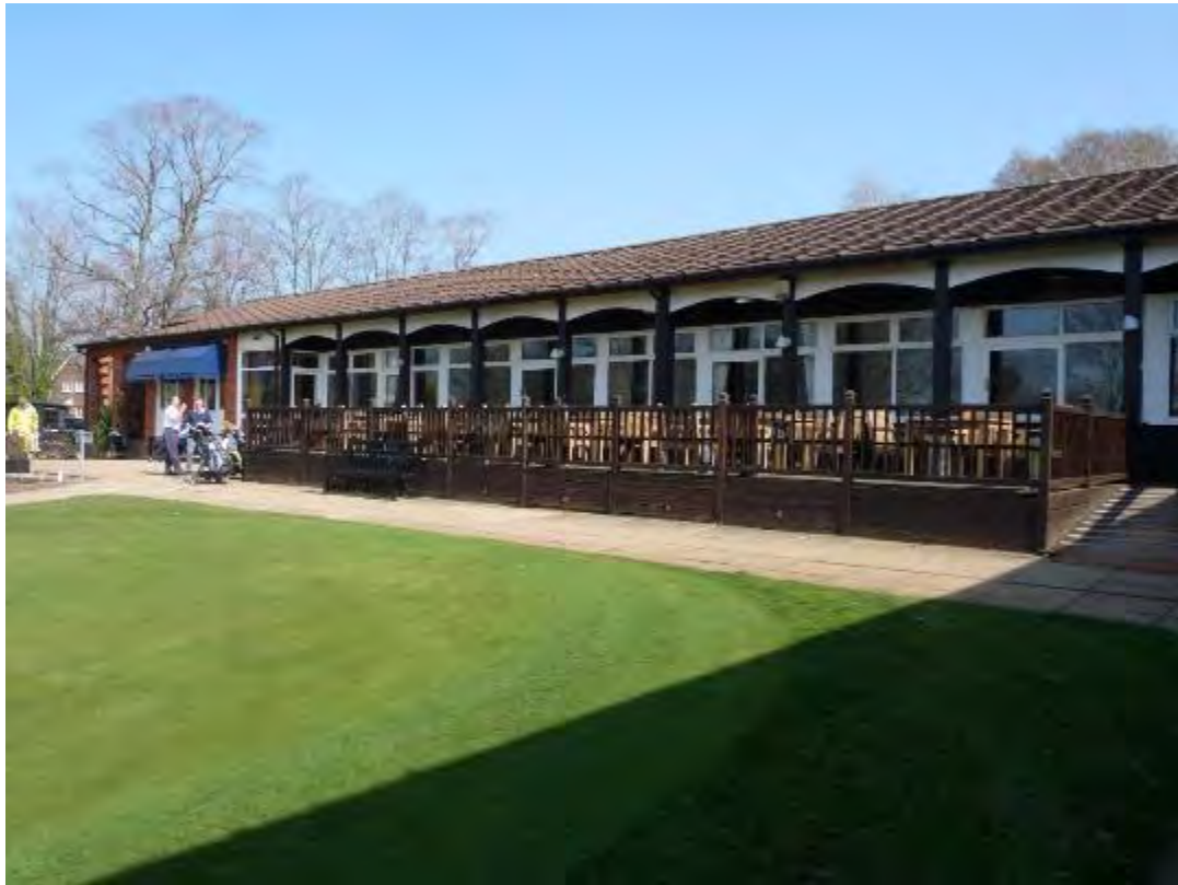
Plate 1: The clubhouse, looking north-east
