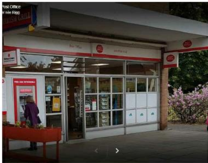
EXISTING SHOPFRONT VIEW
