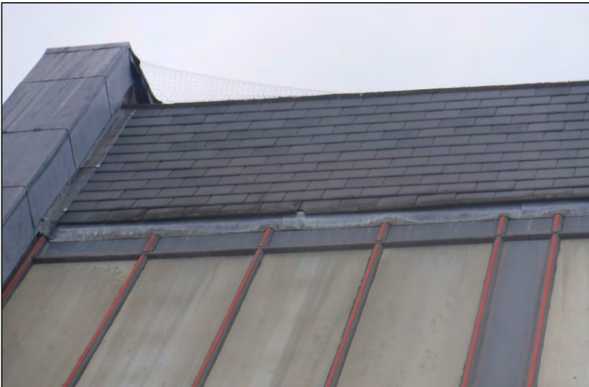
Photograph 7 : Building B1 - Lifted Lead Flashing and Cracked Tile above Glass Atrium
