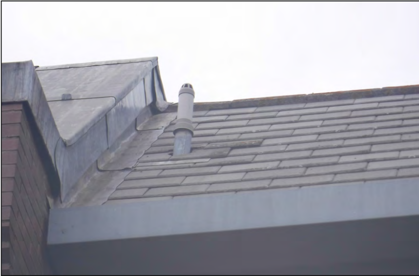
Photograph 7 : Building B1 - Lifted Lead Flashing and Cracked Tile above Glass Atrium
