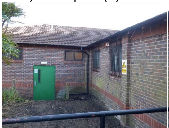
18. Pavilion building with a hipped roof covered in moulded bitumen roof tiles (B1)
