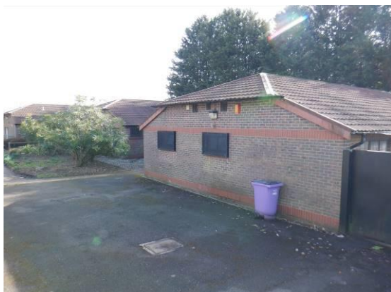
13. Tarmac area at the front (north western) side of the pavilion (OH1)
