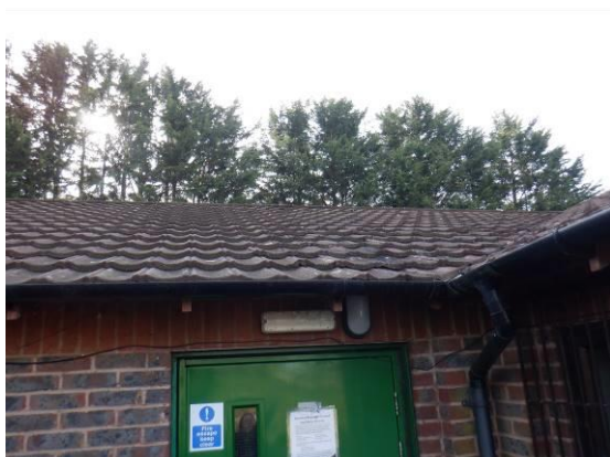
19. Pavilion building with brick walls and a hipped roof covered in moulded bitumen roof tiles (B1)
