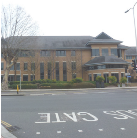
3. Office Building on Vastern Road
