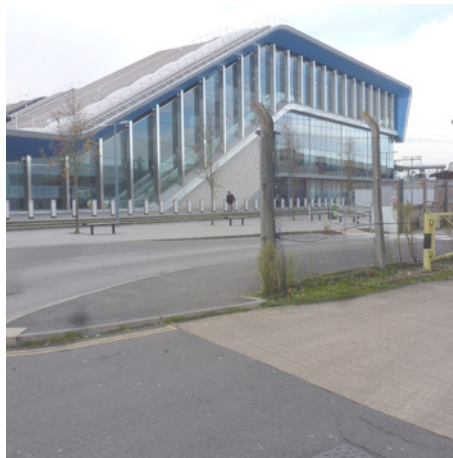
2. Railway station, northern entrance
