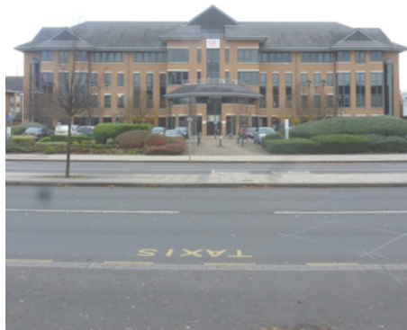
2. Office Building on Vastern Road
