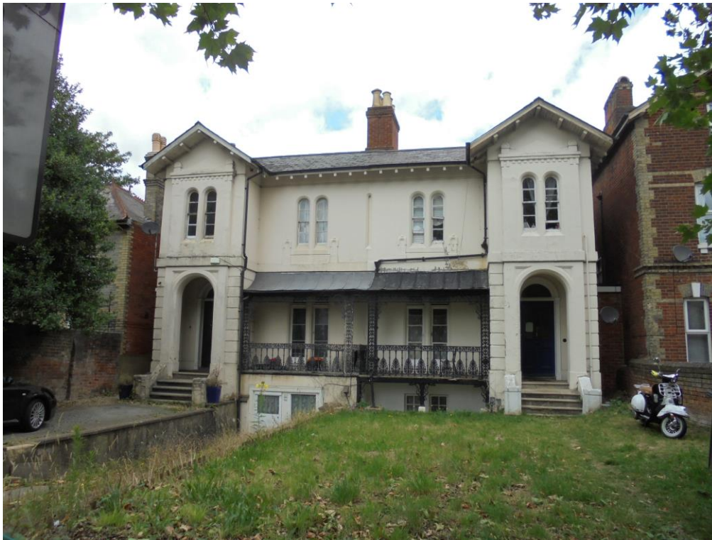
Photo 1 Front elevation of 95/ 97 London Road
