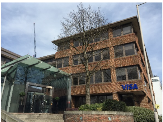
Fig 5: View of the offices building to the NW of the site
