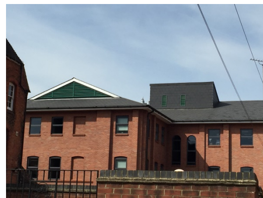
Fig 6: Wall louvre under the gable at the University College of Estate Management
