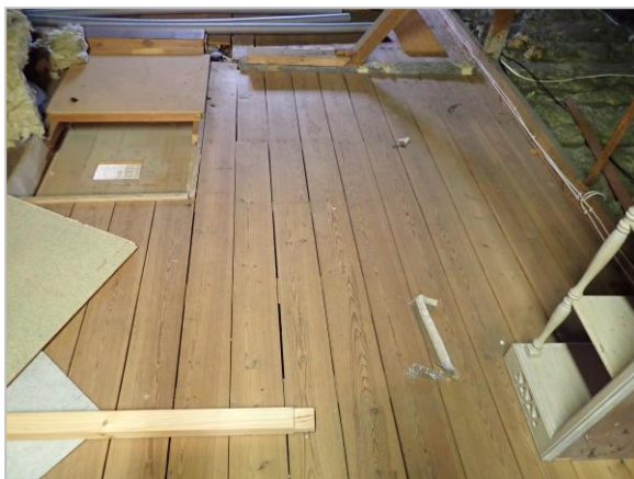
Photo 5 Loft floor boarding
