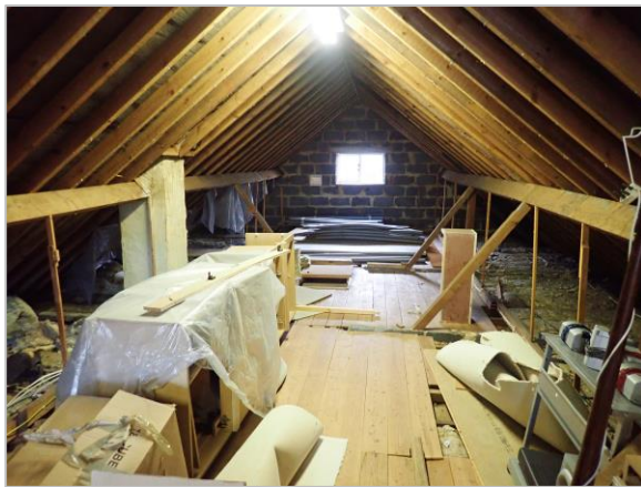
Photo 3 General conditions in loft
