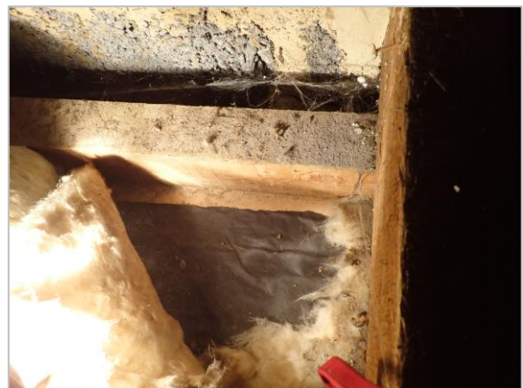
Photo 6 Spot check under insulation
