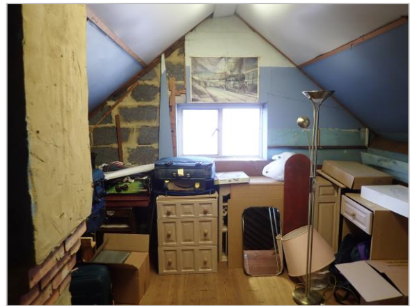
Photo 4 General conditions in loft
