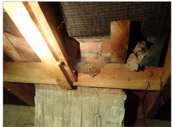
Photo 10 Top of chimney inside loft
