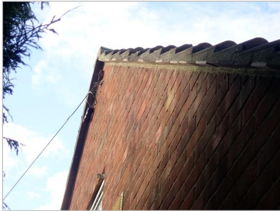
Photo 19 Gable end and verge mortar
