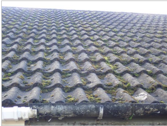
Photo 13 Tiles to front of house
