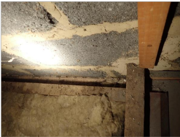
Photo 9 Floor at base of internal gable end wall
