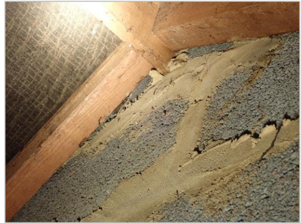
Photo 8 Internal gable apex
