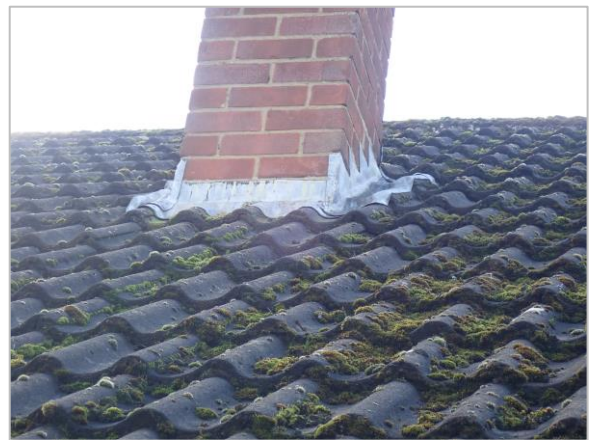
Photo 16 Chimney flashing (rear)
