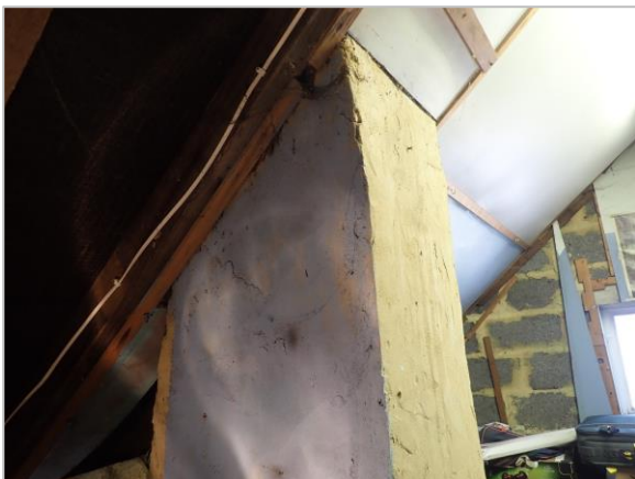
Photo 11 Chimney inside loft
