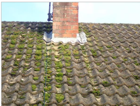
Photo 17 Chimney flashing (front)
