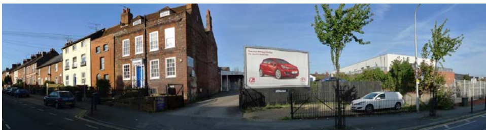
Panoramic view of the site from Mount Pleasant – existing site does not contribute to the urban setting (Advertising sign since removed)
