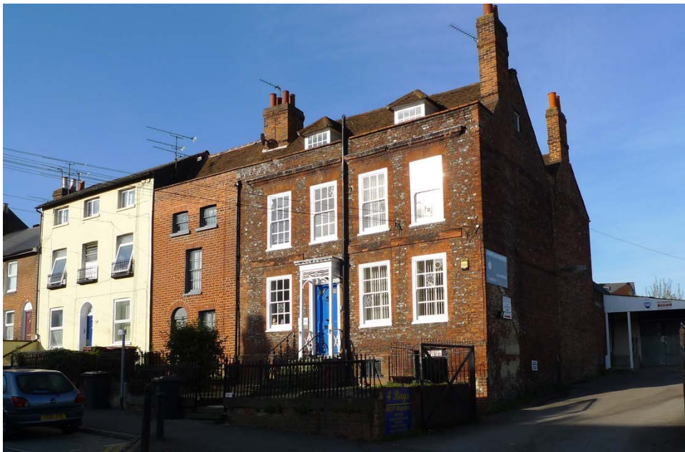
View from Mount Pleasant - No 54, 52 and 50 – listed buildings adjacent to site (left to right)
