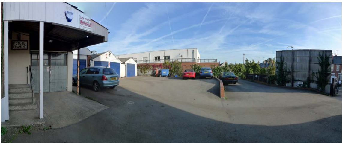
Panoramic view of the site including car repair garages and hard-standing surfaces – the current use is at odds with the residential nature of the area
