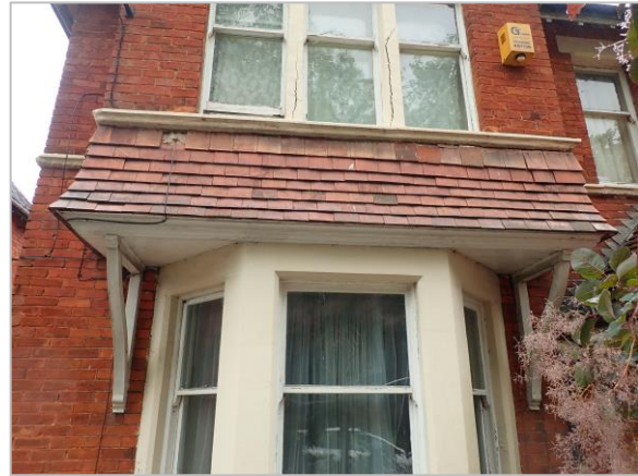
Photo 14 Hanging tiles to front bay
