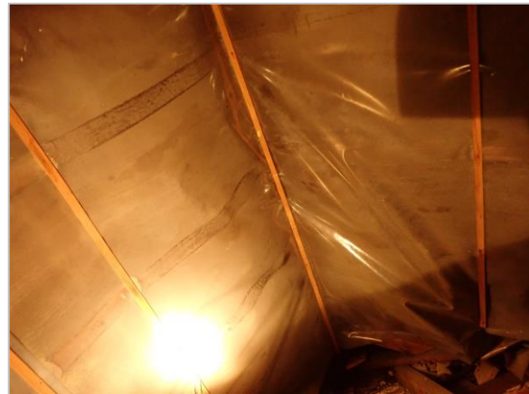
Photo 4 Ridge and internal plastic sheeting
