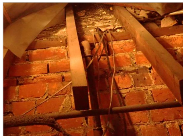
Photo 6 Internal brickwork and timbers
