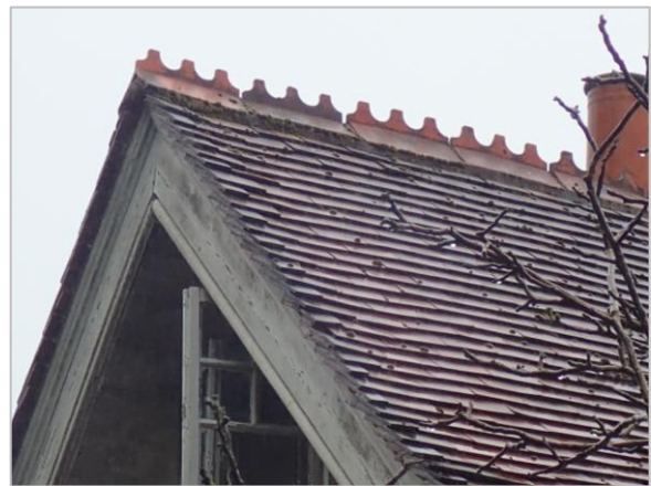
Photo 10 Ridge and bay gable verge
