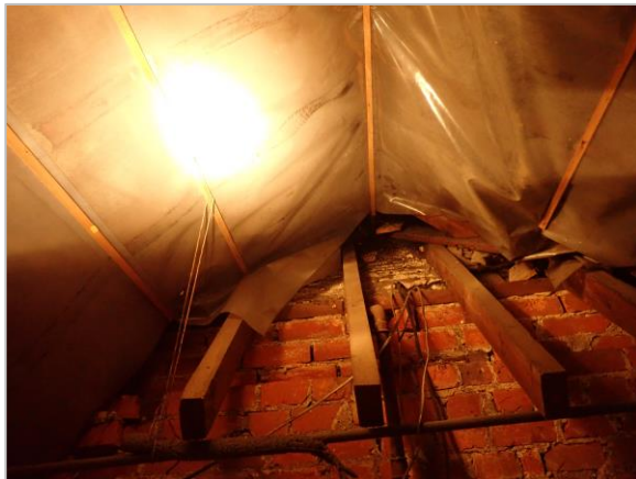
Photo 3 General conditions in loft
