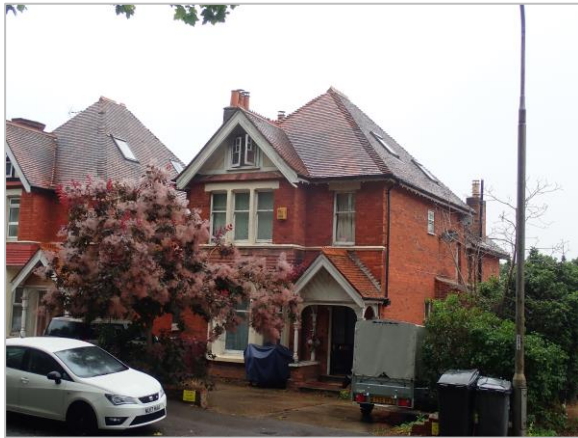
Photo 1 Front (south) elevation
