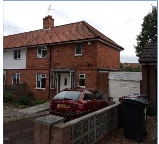
2. Front/Side Elevation of 131 Henley Road (Photo taken on 09/07/2020).
