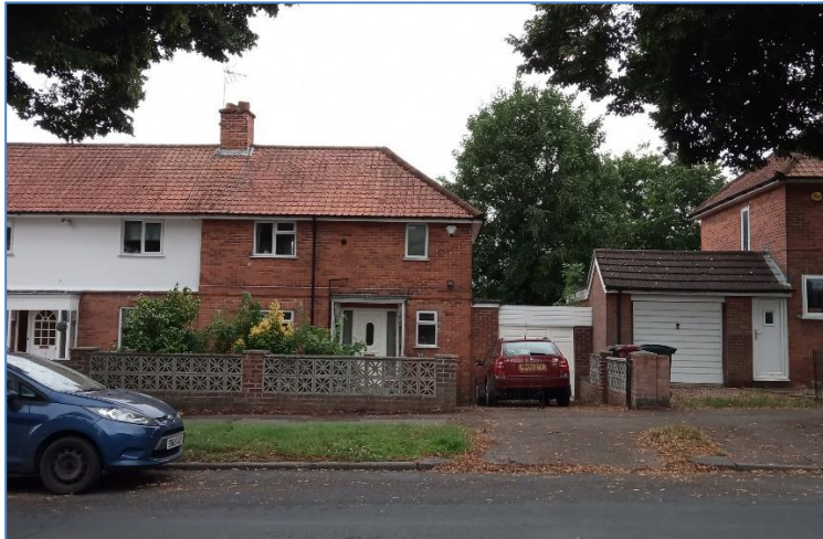
1. Front Elevation of 131 Henley Road (photo taken on 09/07/2020).
