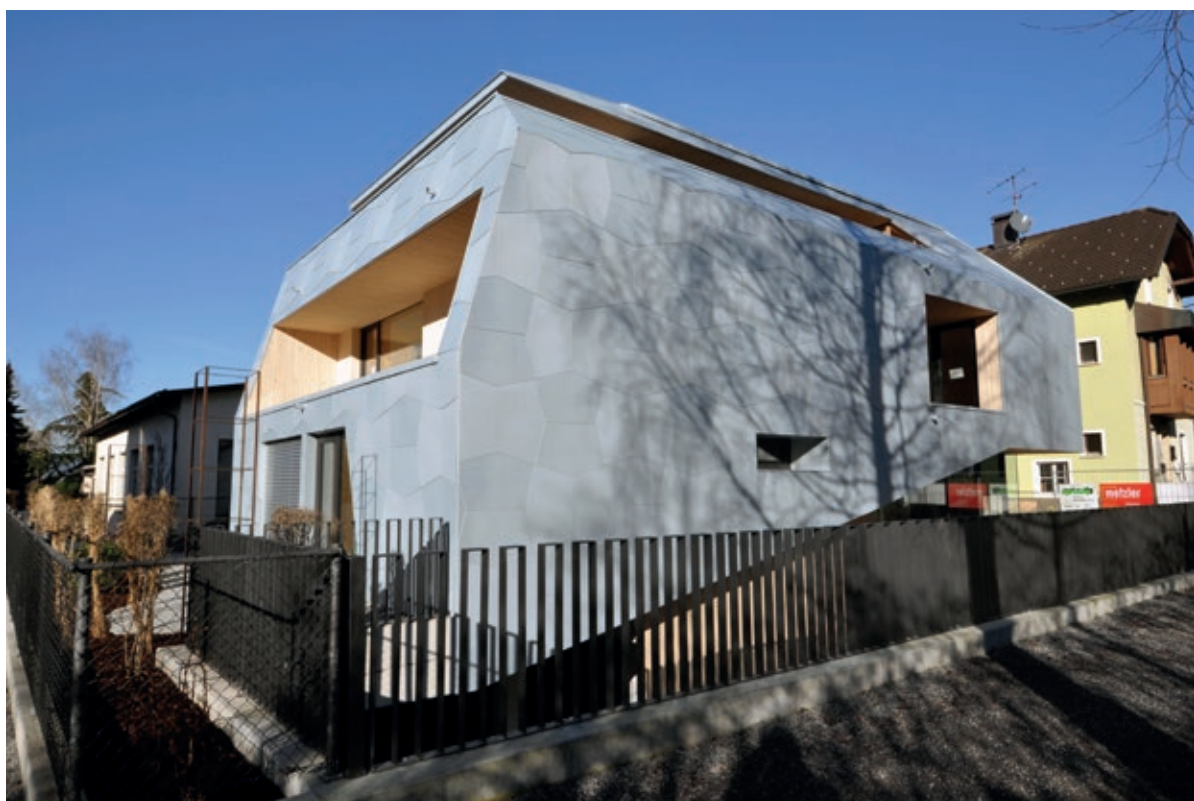
Private House, Hohenems (Austria) Architect: Marc Hoffenscher Aspect: AZENGAR®
