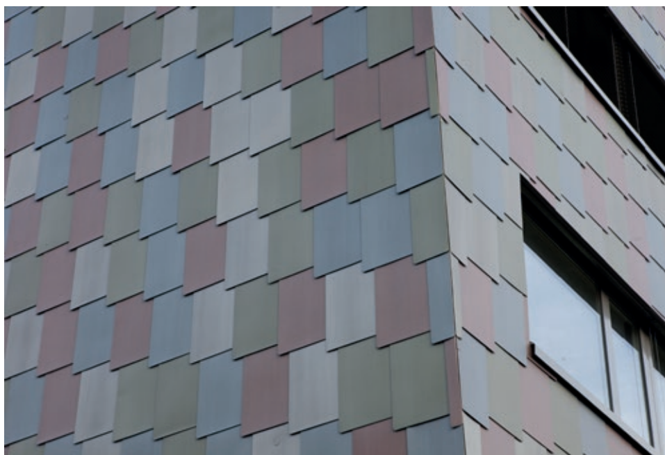
Gare Mittim, Wallisellen (Switzerland) - Architect: CH Architekten AG Volketswil Aspects: QUARTZ-ZINC®, PIGMENTO® red, green, blue
