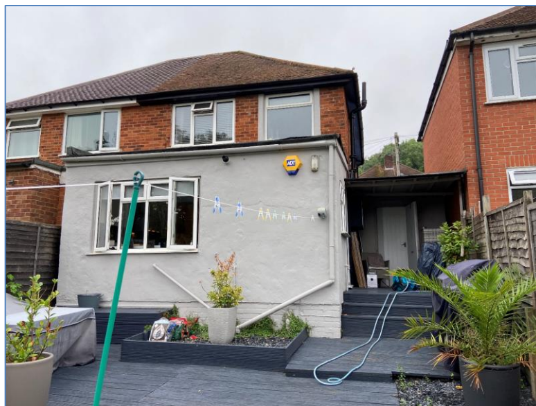
1. Rear of 44 Coniston Drive. Photo provided by the agent on 11/10/2020.
