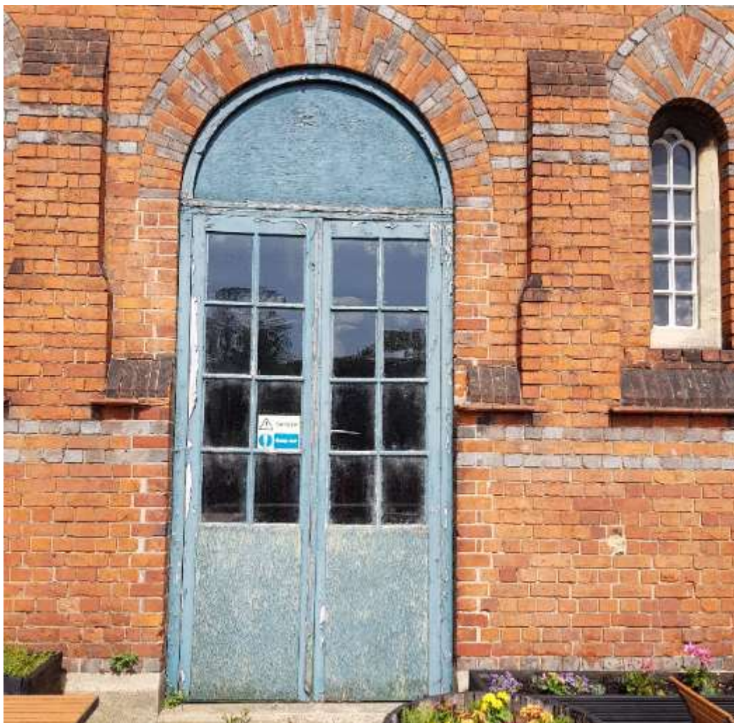
Photograph 1: Existing doors on south elevation.
