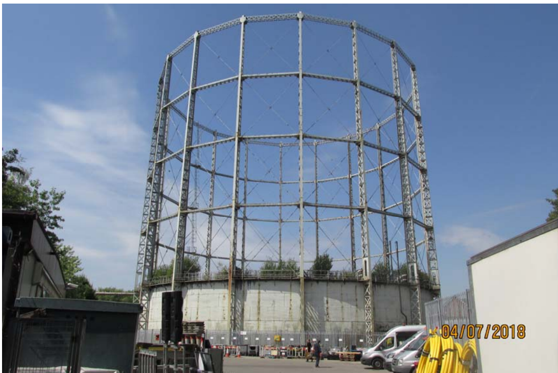
Plate 2. Gasholder located within the site
