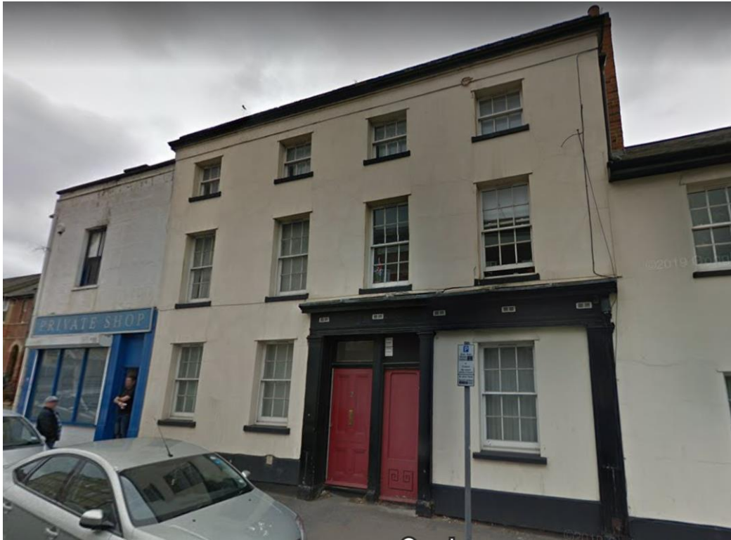
Front (east) façade of 106 Southampton Street
