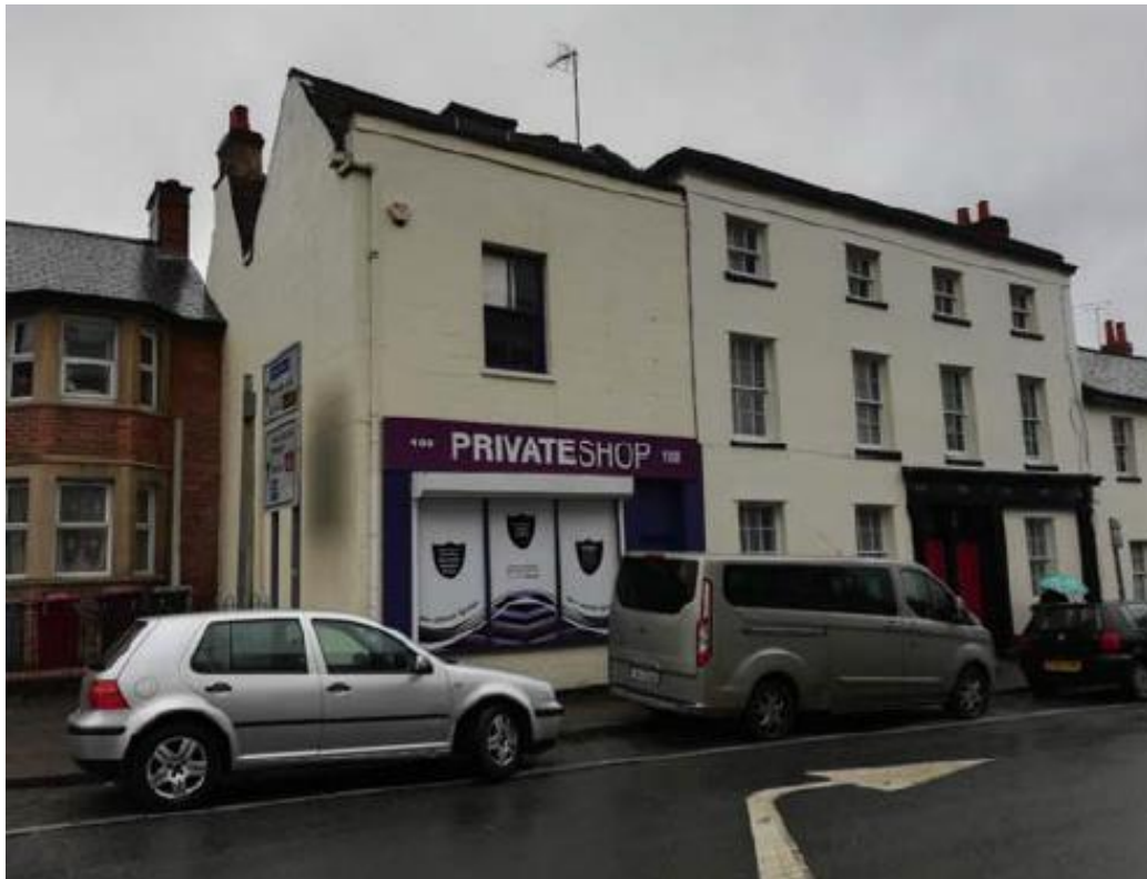
Front (east) elevation of 108 Southampton Street
