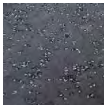
Carriageway New and Existing made good) tarmac
