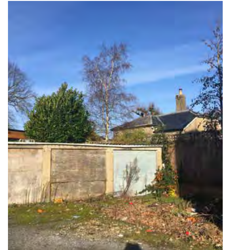
10 - View of existing garages (Looking north-east)
