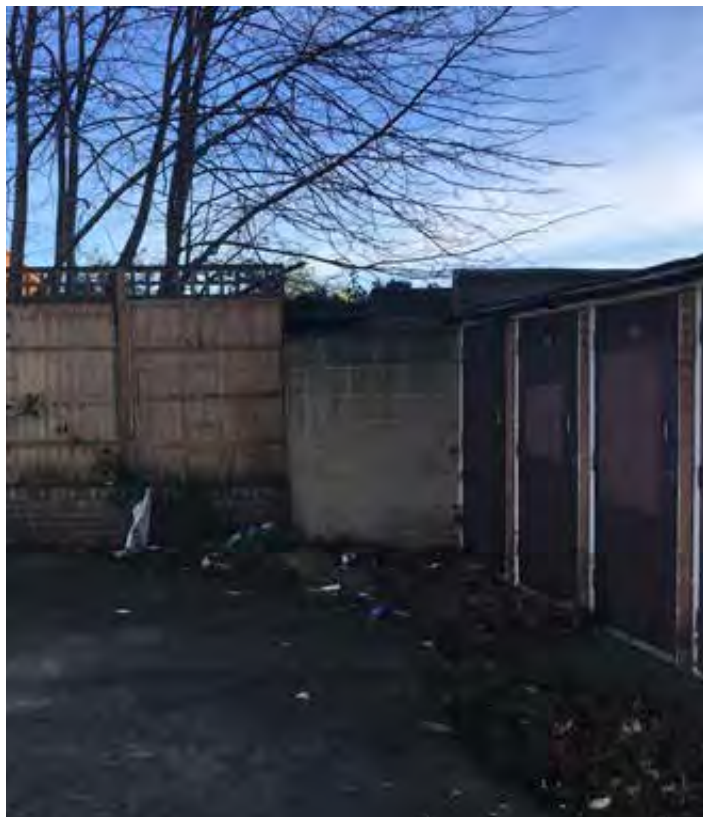
11 - View to eastern boundary
