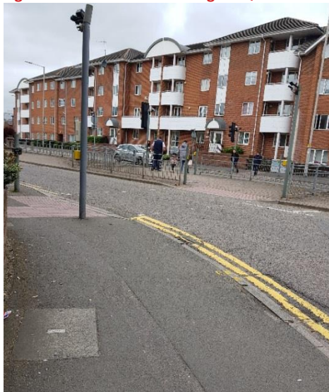
Figure 2.5. Signalised Pedestrian Crossing on Queen's Road
