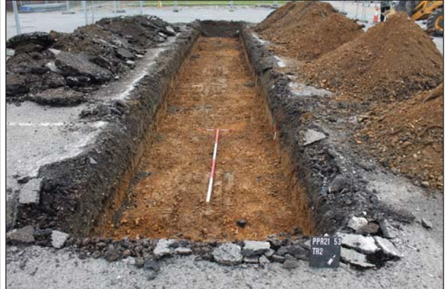
Plate 2. Trench 2, looking south-east, Scales: 2m and 0.5m.
