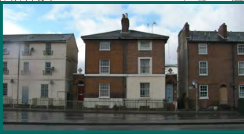
29 and 31 Caversham Road (Grade II)
