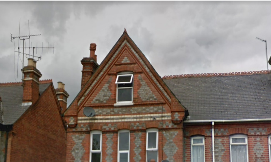
4. Oxford Road Houses - Recessed brick work
