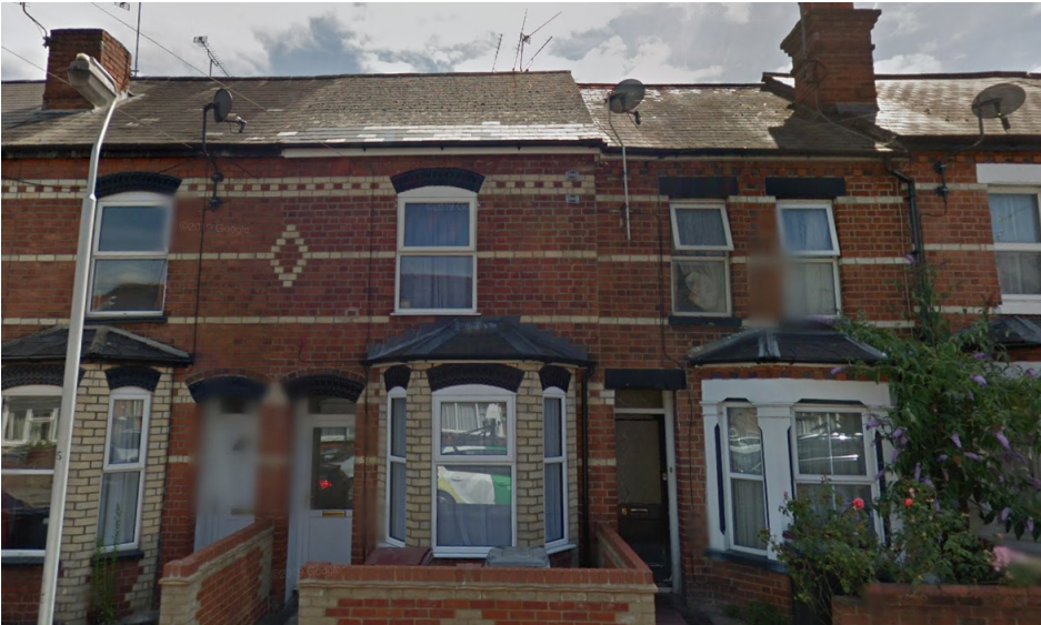
3. Nearby Terrace Housing - Feature brick banding
