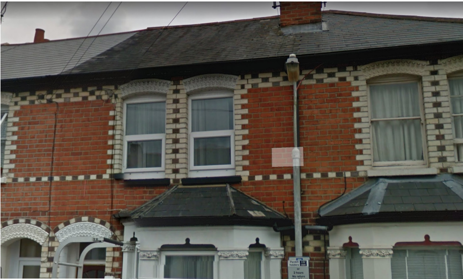
2. Nearby Terrace Housing - Feature brick banding
