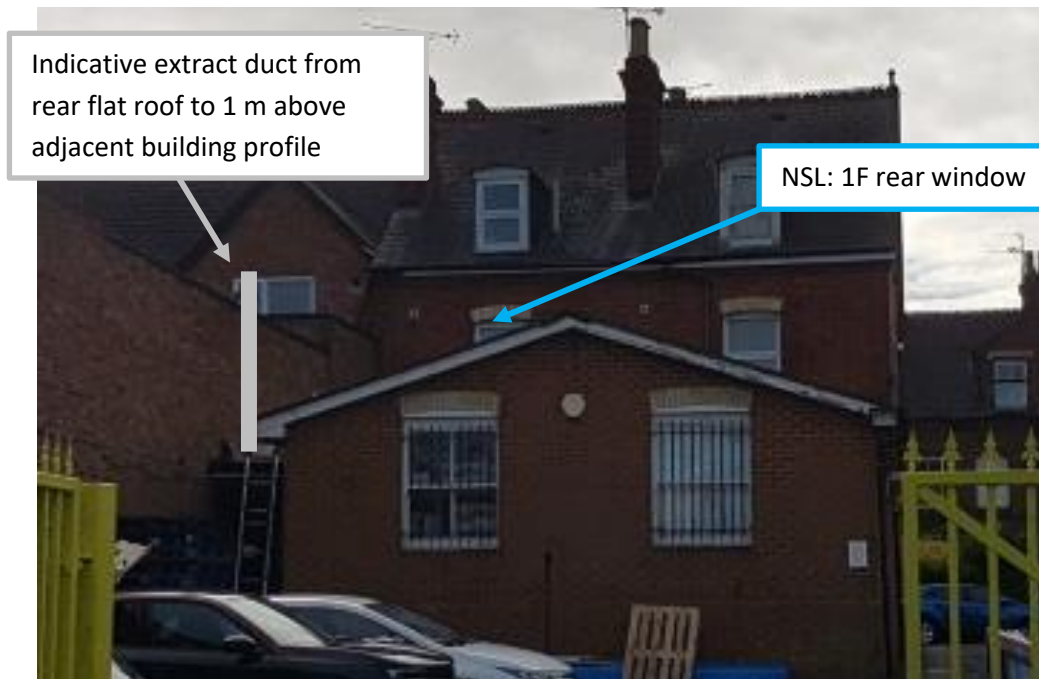
Figure C2 – Photo showing rear of The Site with indicative extract ducting location and nearest noise sensitive location annotated.
