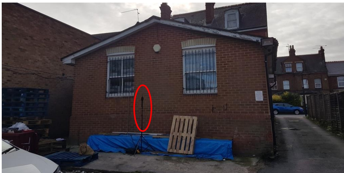
Figure D1 – Photo highlighting measurement Position 1, rear of site 734 - 736 Oxford Road.
