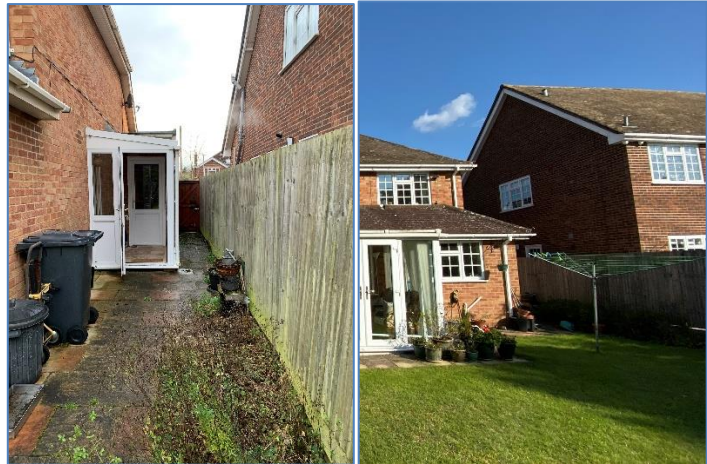
Fig 5. Existing side elevation in relation to 6 Highdown Hill Road. Site photo provided by agent on 22/12/2020.
