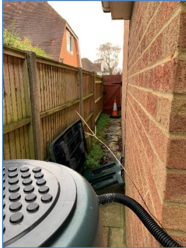
Fig 4. Existing side elevation in relation to 8 Highdown Hill Road. Site photo provided by agent on 22/12/2020.
