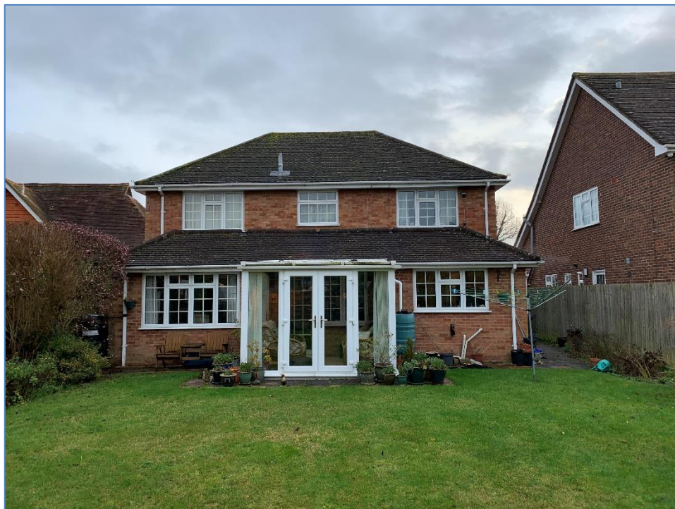
Fig 1. Rear of 6a Highdown Hill Road. Site photo provided by agent on 22/12/2020.
