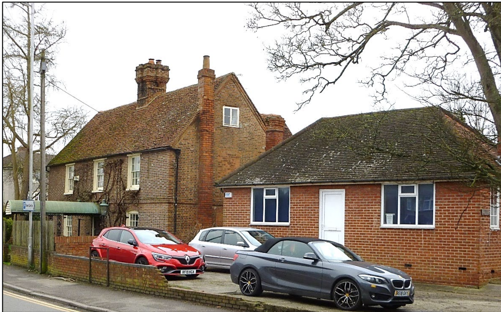
Plate 3: View of the Site's frontage and Ivy Farmhouse from the northwest
