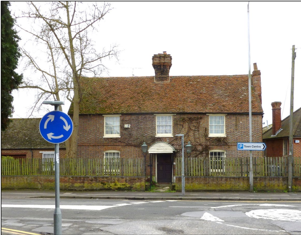
Plate 1: Front (northern) elevation of Ivy Farmhouse
