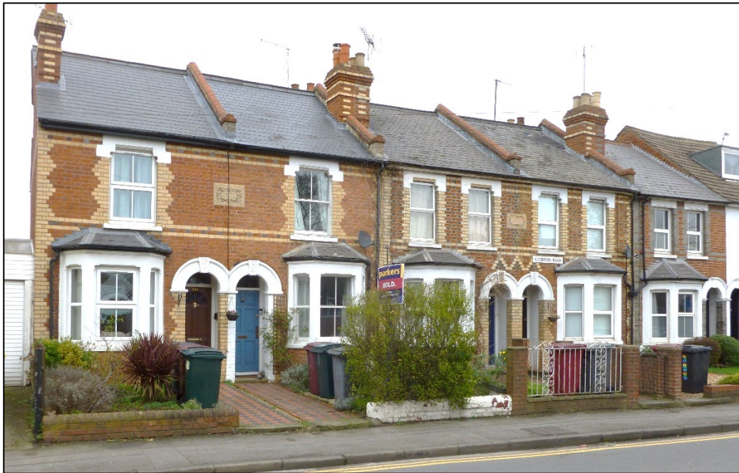
Plate 5: View of Victorian brick-built terrace on Gosbrook Road to the north of the Site
