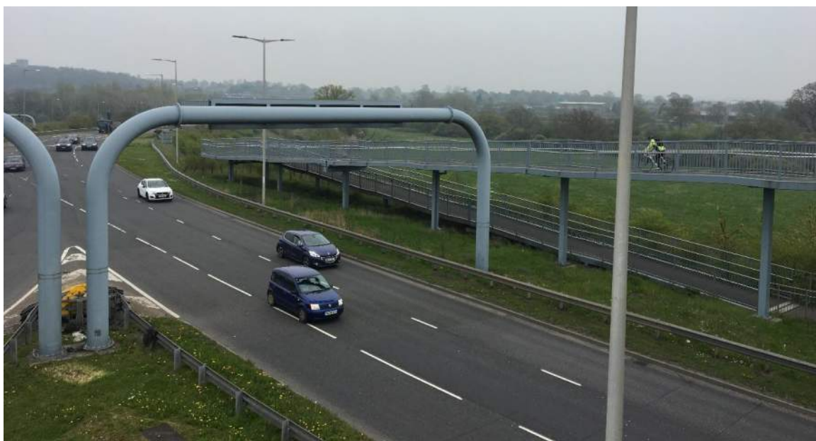
Figure 2–9: Cycle ramp across the A33
