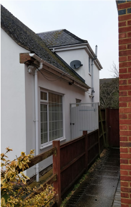
Image 3. Side elevation of neighbouring house
