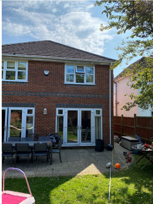
Image 8. Rear elevation, south west boundary
