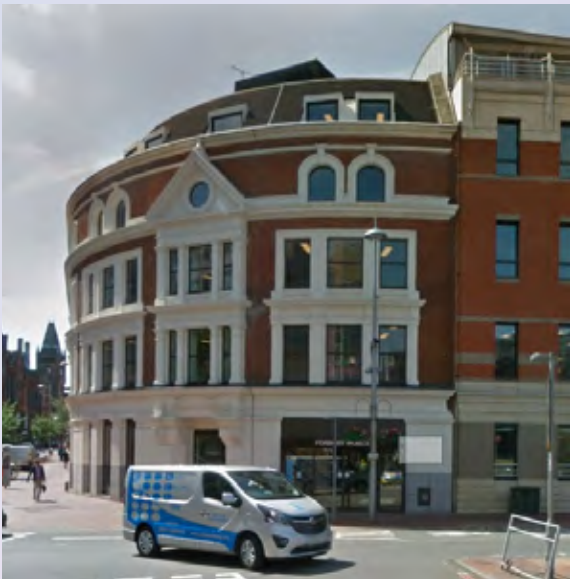
Forbury Works, Blagrove Street
