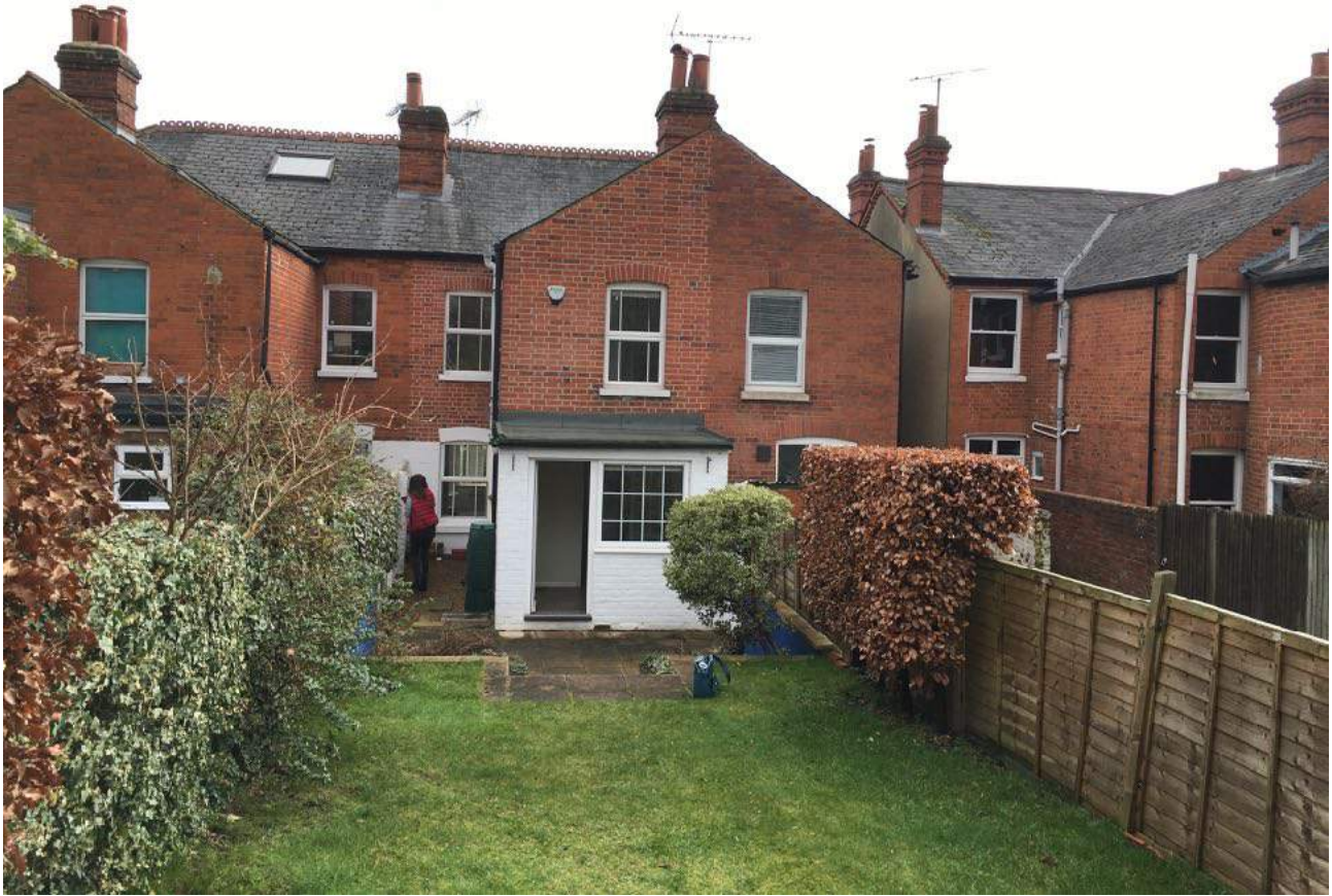
Photograph showing rear elevation of the property
