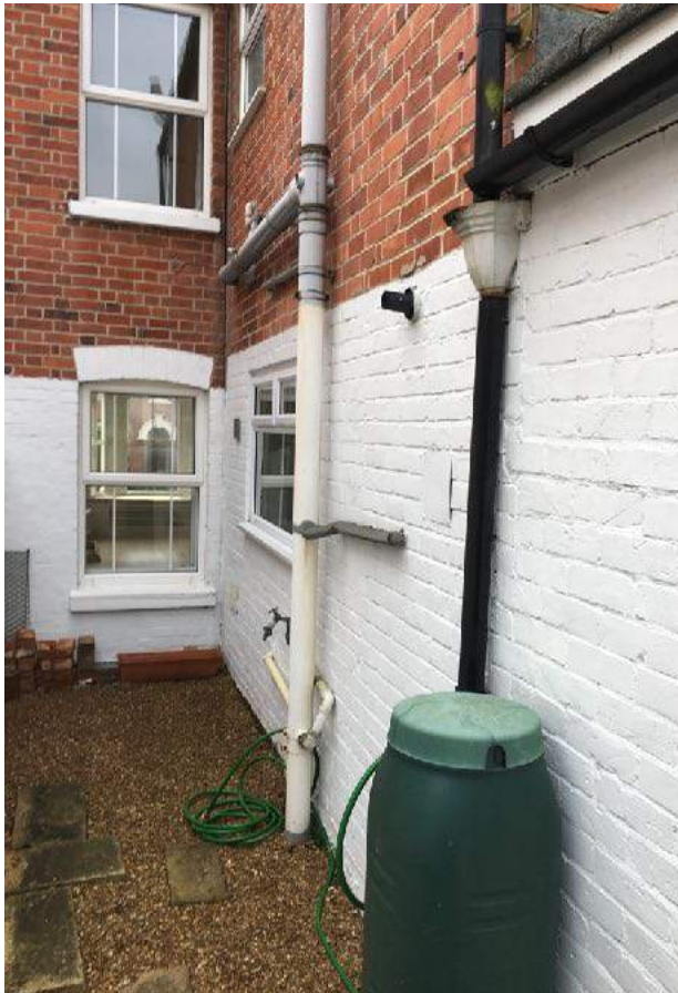
Photograph showing existing passage area to the rear and brickwork boundary wall
