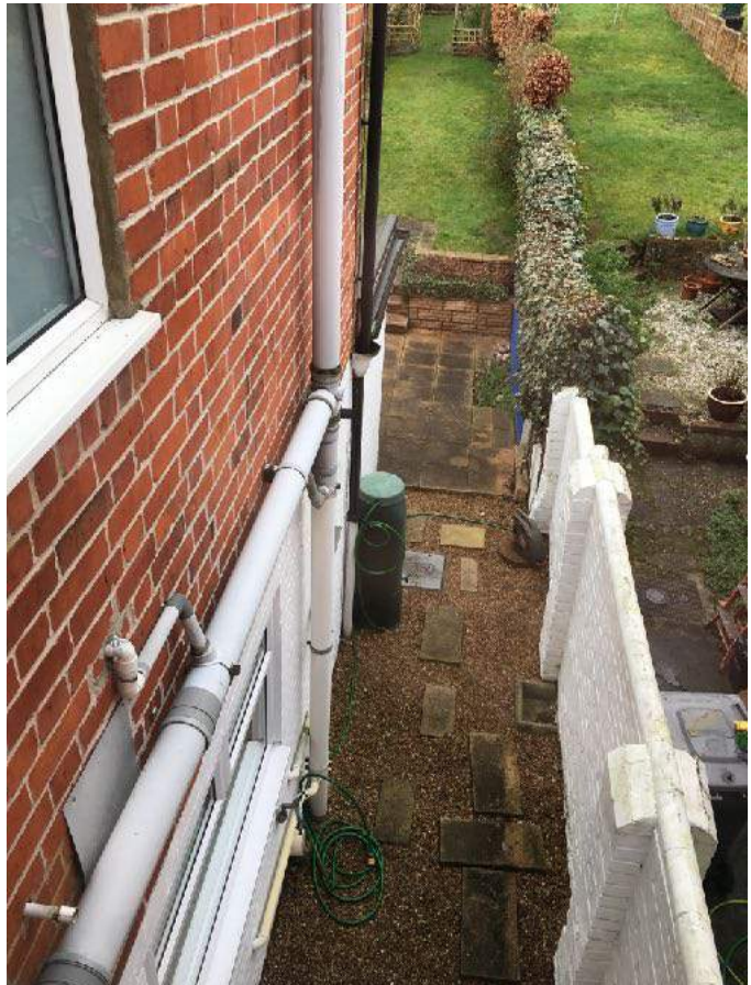
Photograph from first floor of the property showing existing passage area to the rear and brickwork boundary wall
