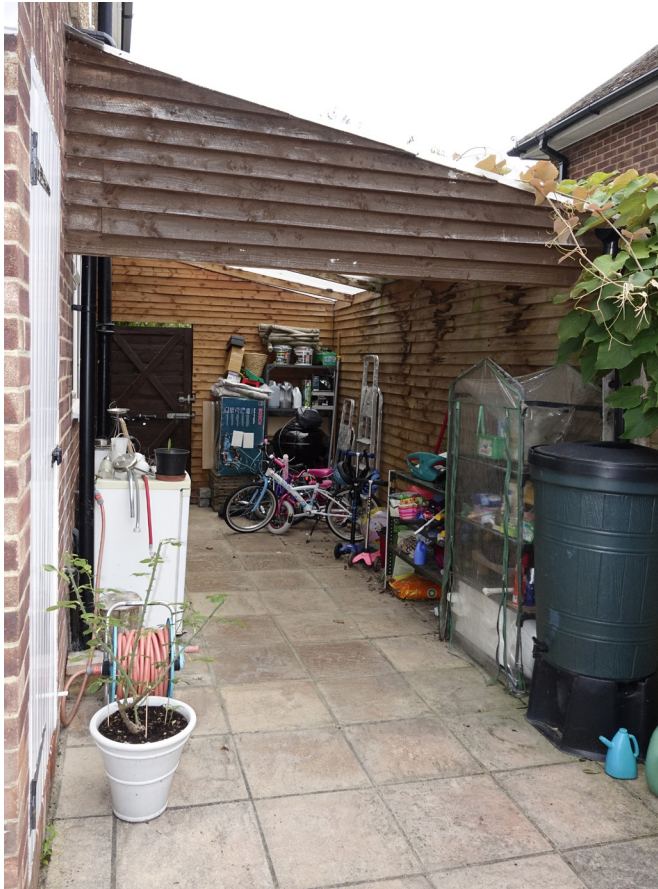
Lean-to as viewed from rear
