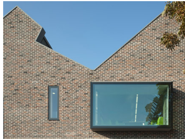
Below: Precedent studies illustrating examples of material & colour palettes; From LtoR: Brick features; Contemporary gable end house with red/grey brick and dark joinery with thin roof edge detail; Brick feature details with dark joinery & thin roof edge profile; Dark brick with timber cladding & dark joinery
