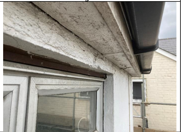
Photo 8 Sealed soffit
