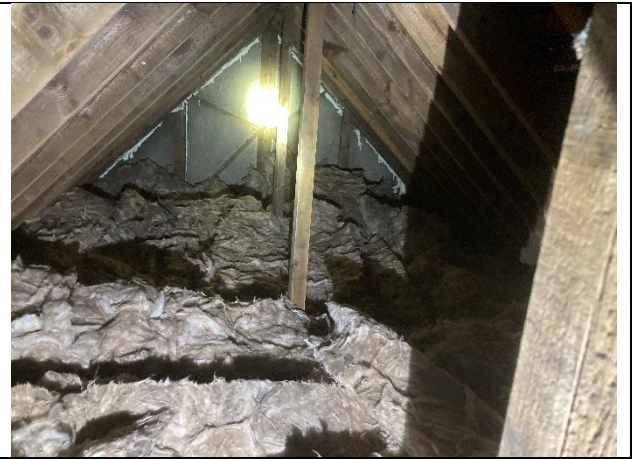
Photo 6 West interior gable
