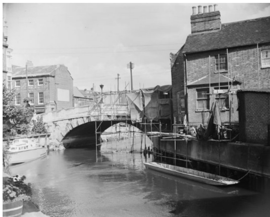
Figure 4.7 High Bridge in 1951 (Source: Reading Museum online, published by Berkshire Chronicle on 13 September 1957)
