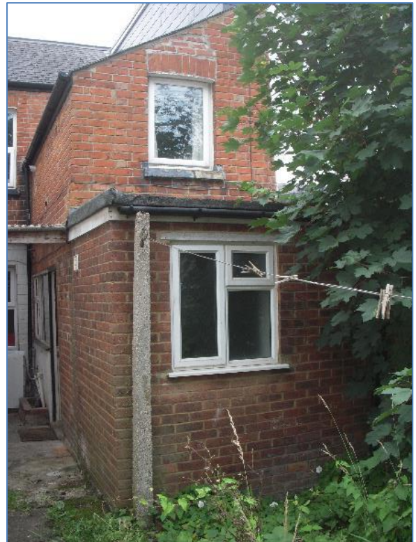
2. Rear of 3 Hatherley Road. Photo provided by the agent on 25/08/2020.
