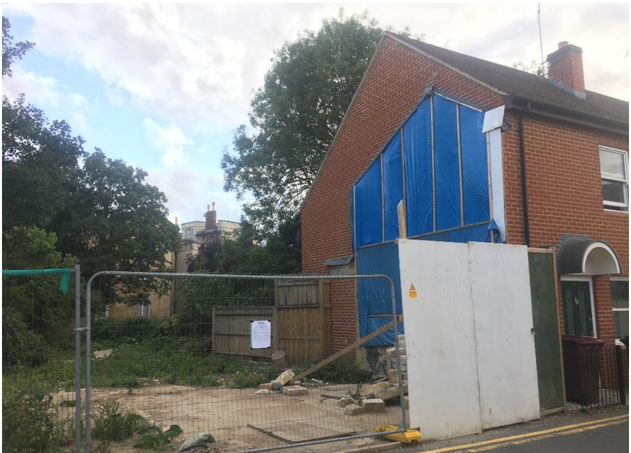
Site photograph provided by the applicant on 21/08/2020
