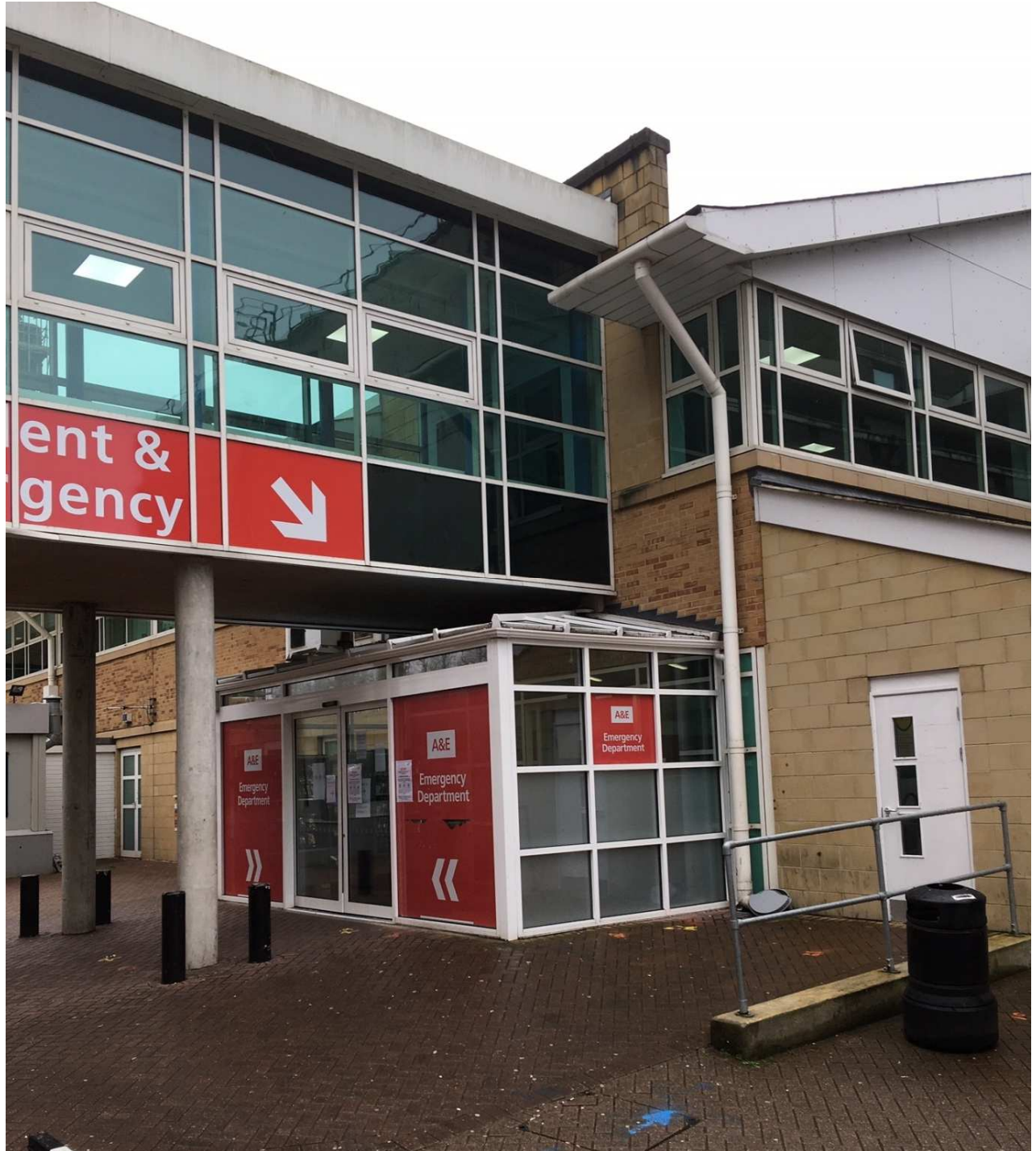
Figure 6: View of Existing A&E entrance looking from the northwest.
