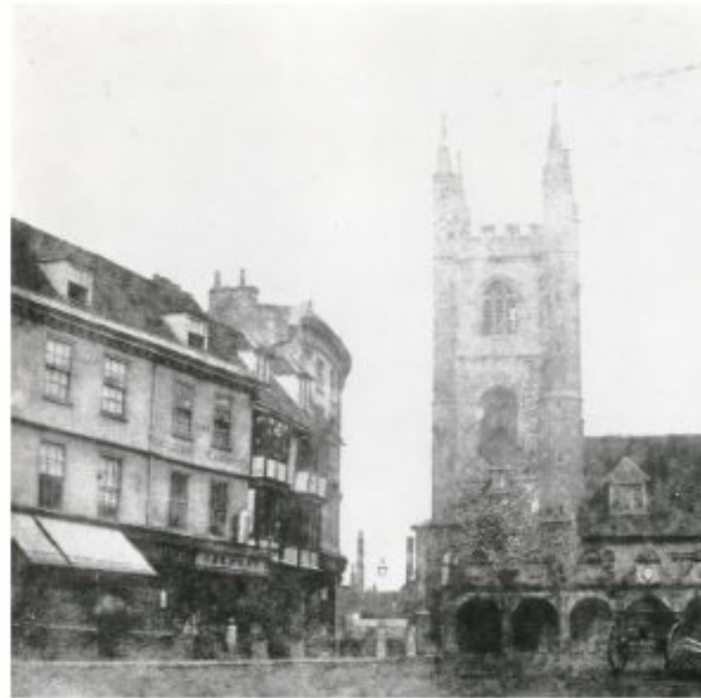
A view from Market Place of St. Laurence Church. The application site is the Listed buildings to the left in the photo.
