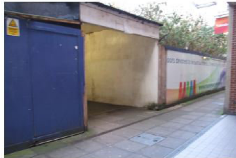
The rear entrance of the arcade opposite Sainsburys
