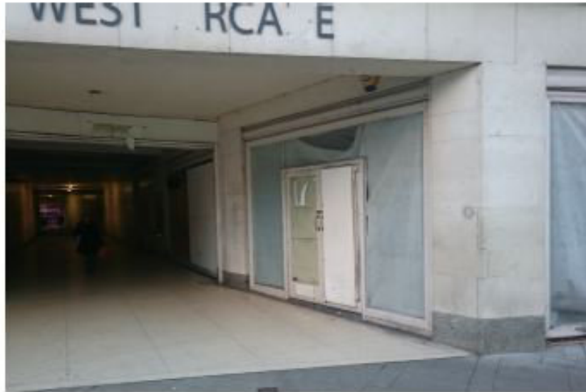
A view of the front of the arcade on Town Hall Square.
