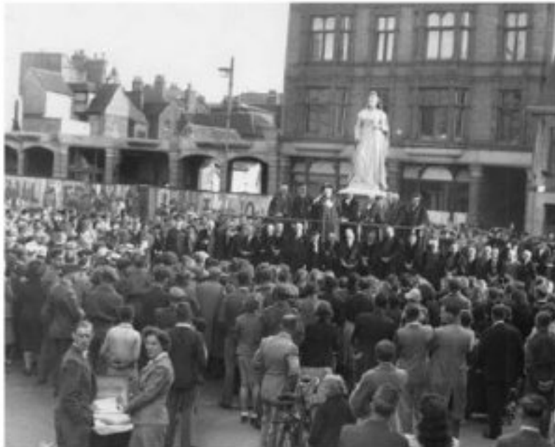
View of the partly demolished arcade building following WW2 bomb damage.
