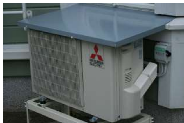
Figure 4: Outdoor unit of an ASHP.
