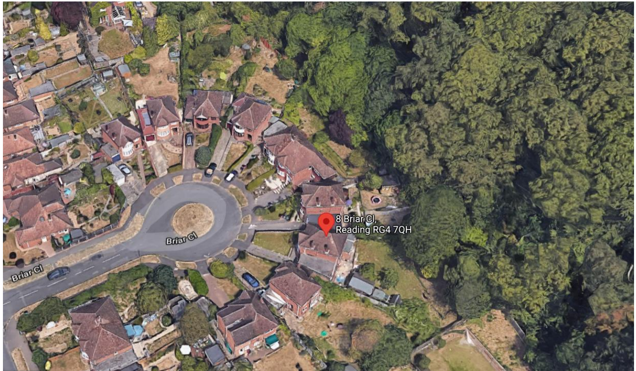
Aerial view looking north
