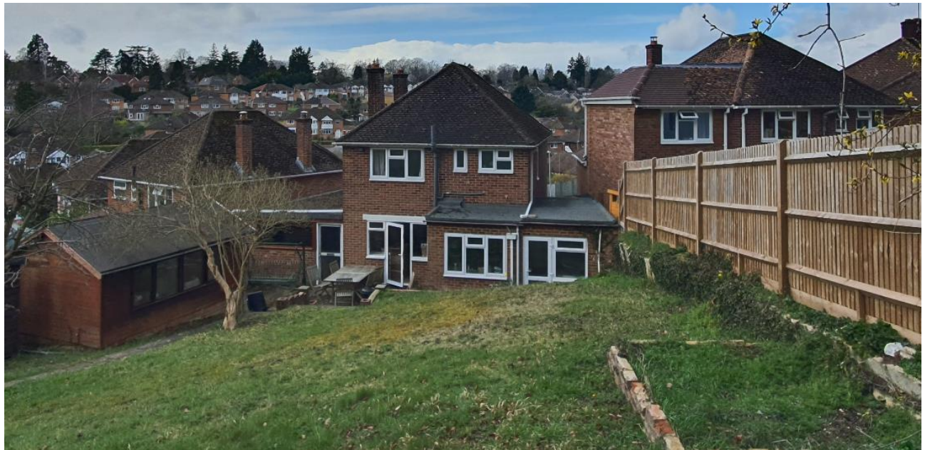
Rear garden/elevation (photograph provided by the applicant)
