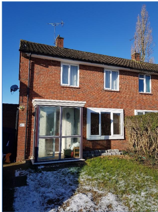
1. Front of 25 Warnford Road. Photo provided by the agent on 05/03/2021.
