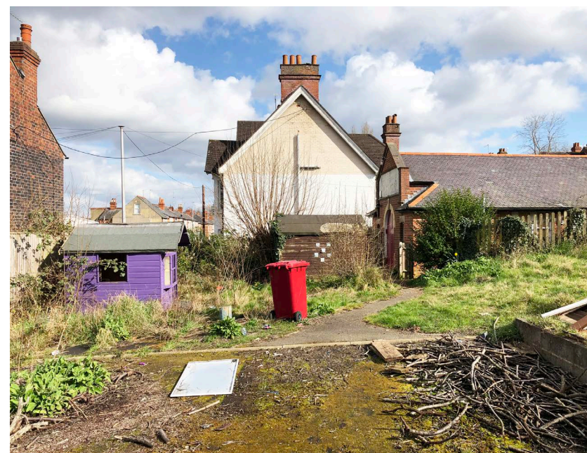
2. Looking West at side elevation of 57 Gloucester Road
