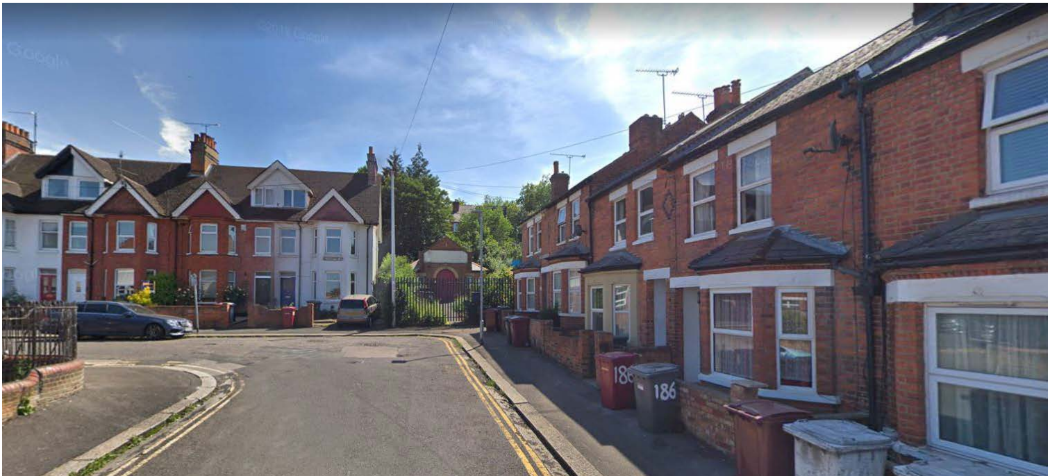
2.2 2 and 3 storey Victorian terraces on Gloucester Road and Kensington Road
