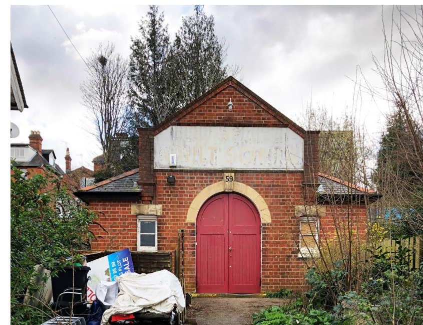
6. Existing studio on site (North facade)
