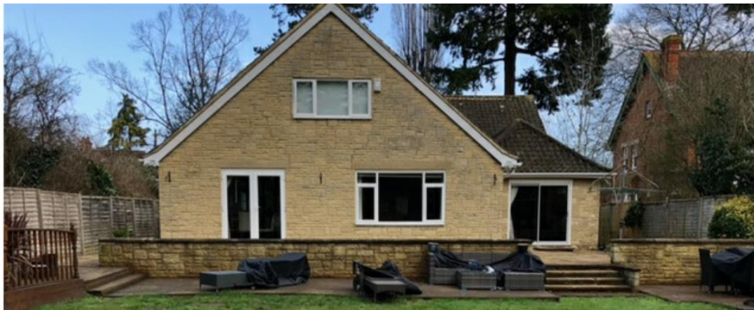
Rear of 19 Conisboro Avenue
