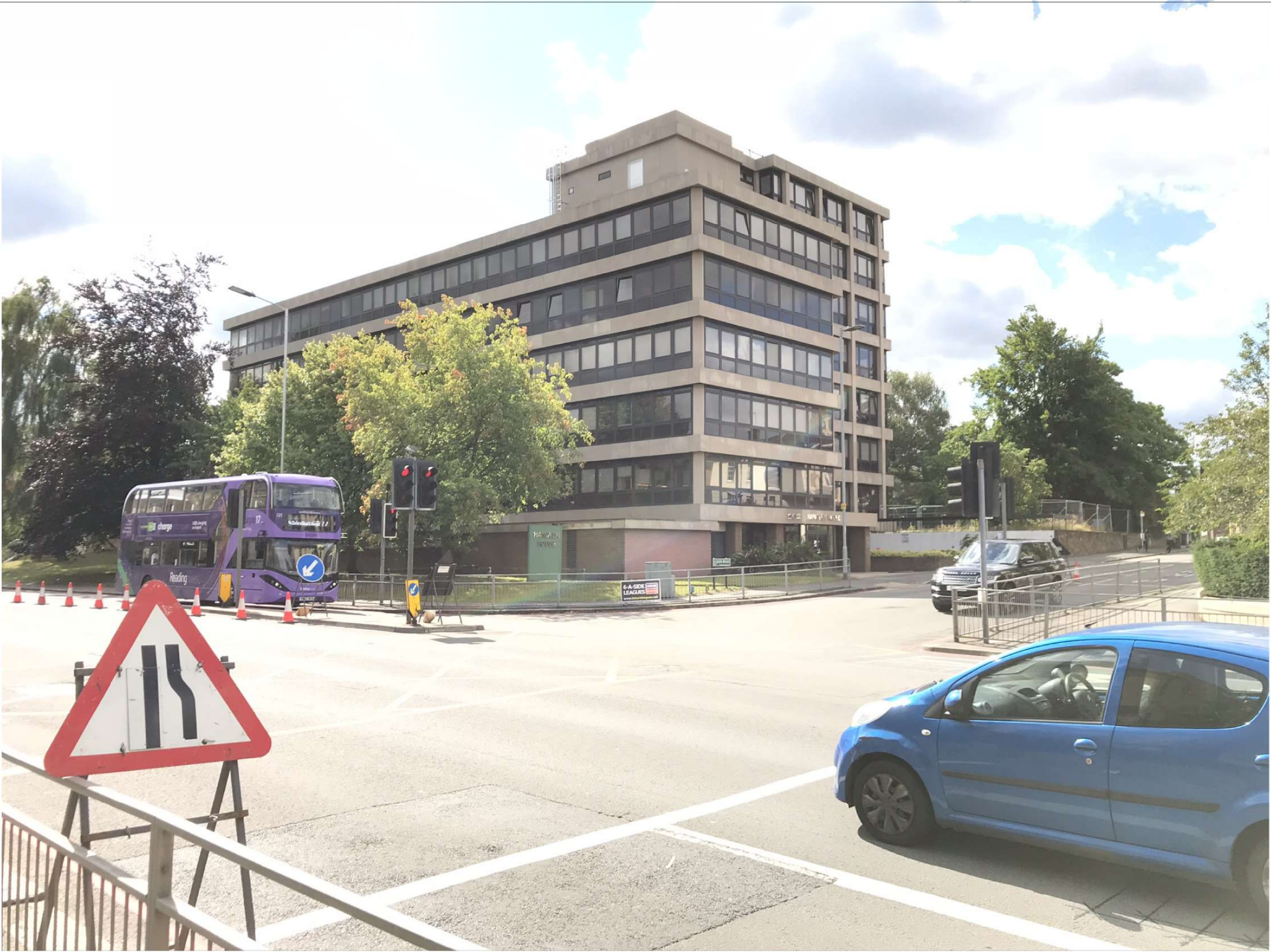
Existing Building - View from King's Rd
