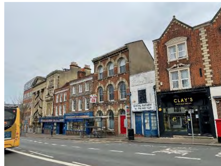
Plate 12: The east side of London Street and the site when viewed from further south.
