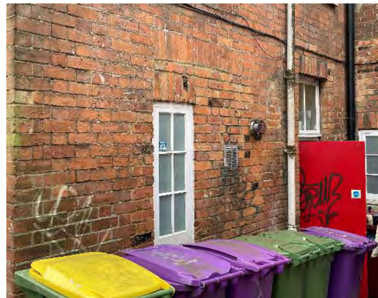
Plate 22: Modern window and infill brickwork with the historic arch still visible.
