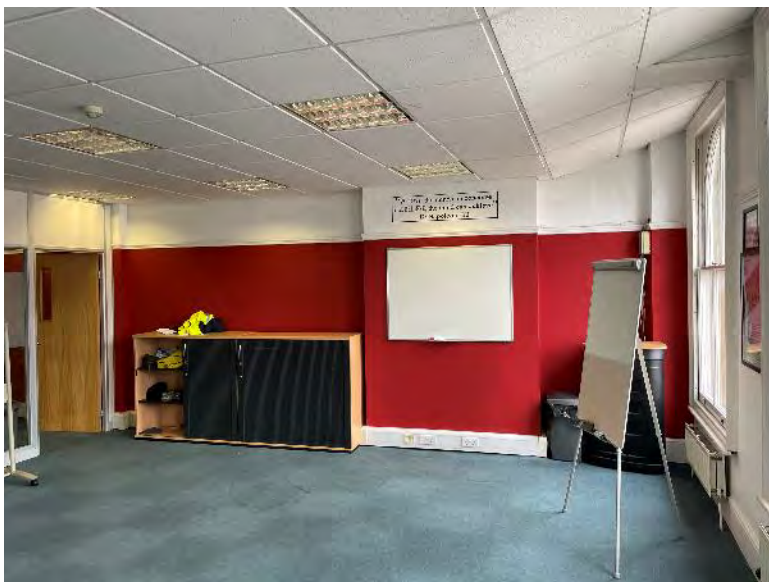
Plate 24: Single room at first floor level with the chimney breast visible.
