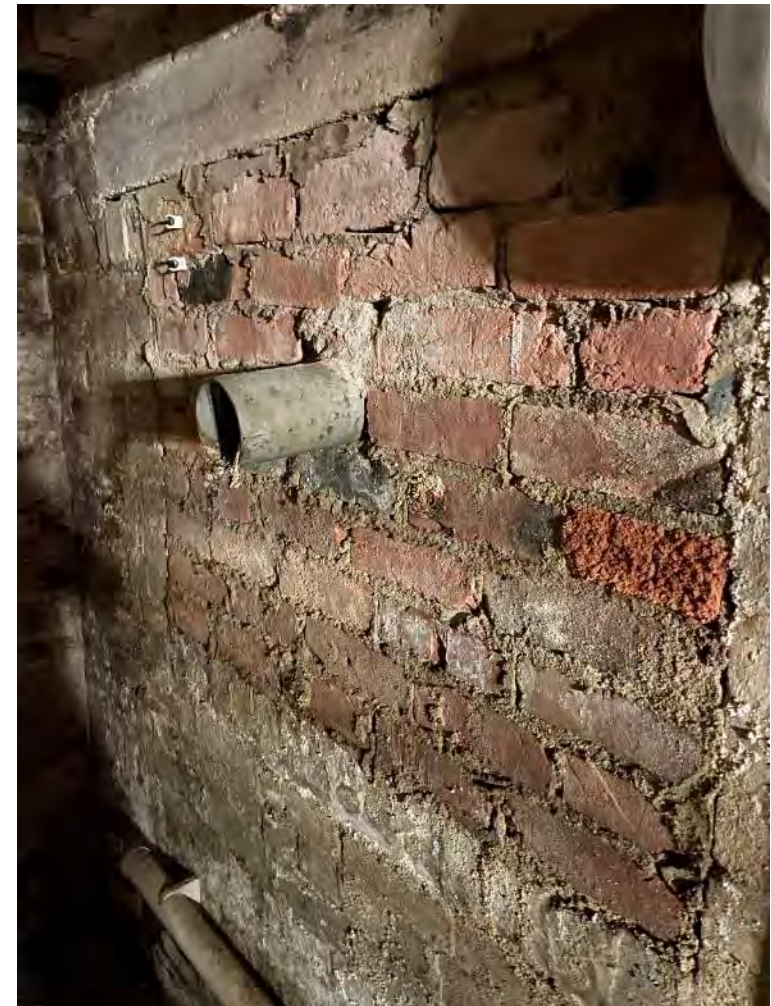
Plate 19: Blocked up coal shoot at basement level.
