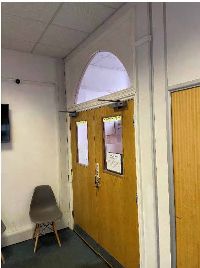
Plate 15: Existing ground floor entrance from the hall.
