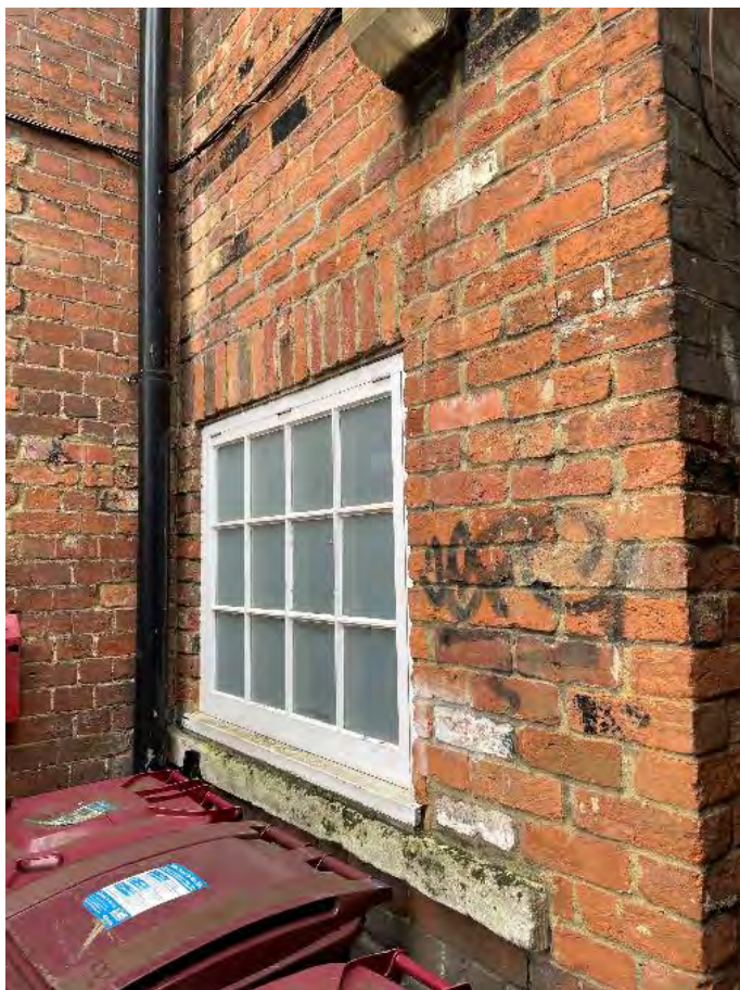
Plate 20: Modern window with infill brickwork. Historic sill remains.
