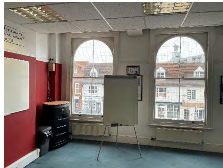
Plate 14: Existing first floor finishes.
