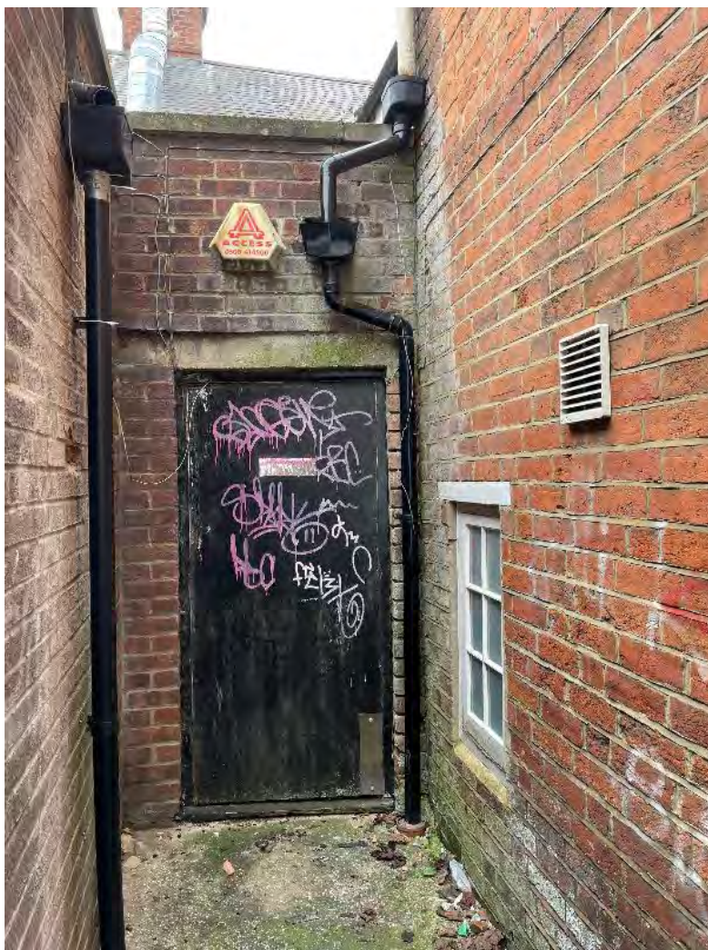
Plate 23: Modern window to be removed.
