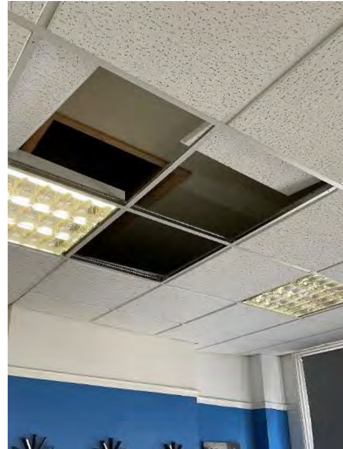
Plate 26: Modern ceiling fabric and structure behind the suspended ceiling.
