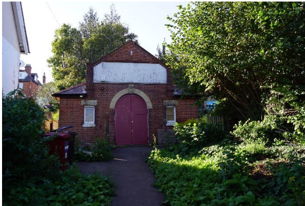
Photograph 1. The building at 59 Gloucester Road.
