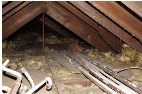
Photograph 2. The loft space of the building.
