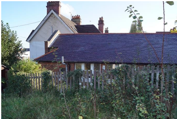
Photograph 3. The building viewed from the west.
